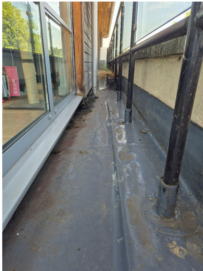
View of the parapet
