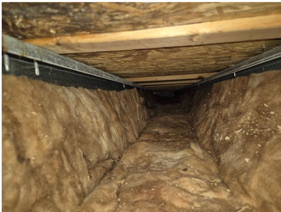
View within the roof void. Note minimal supporting structure to the terrace decking.
