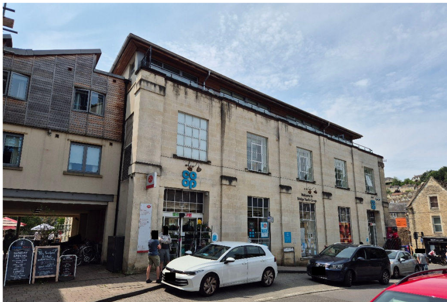
View of the North East elevation of the property taken from Bridge Yard
