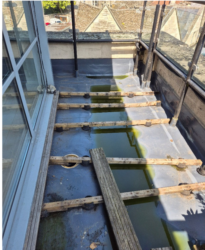
View of a roof terrace area
