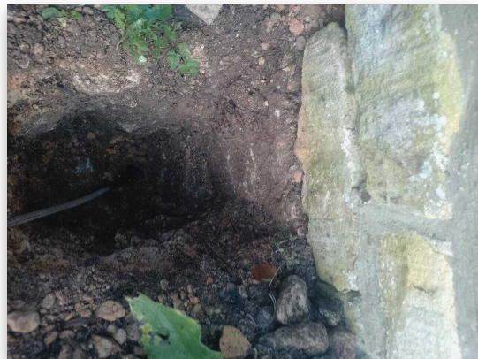
Fig 1.2: Trial Hole 1 Footing
