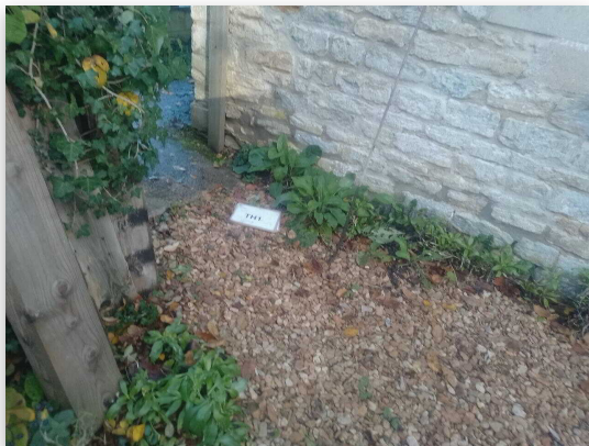
Fig 1.1: Trial Hole 1 Location
