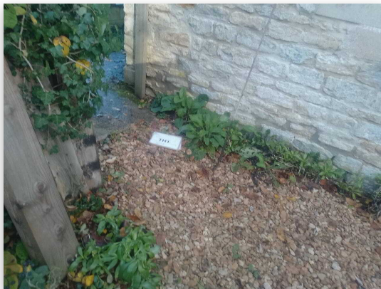
Fig 1.1: Trial Hole 1 Location
