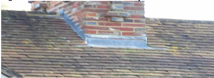
Figure 8/9. Leadwork around chimney.
