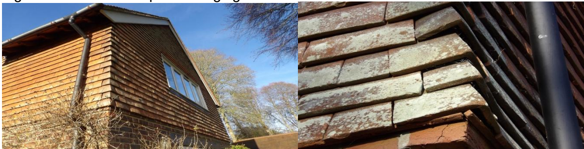
Figure 10/11/12. Example of hanging tiles.
