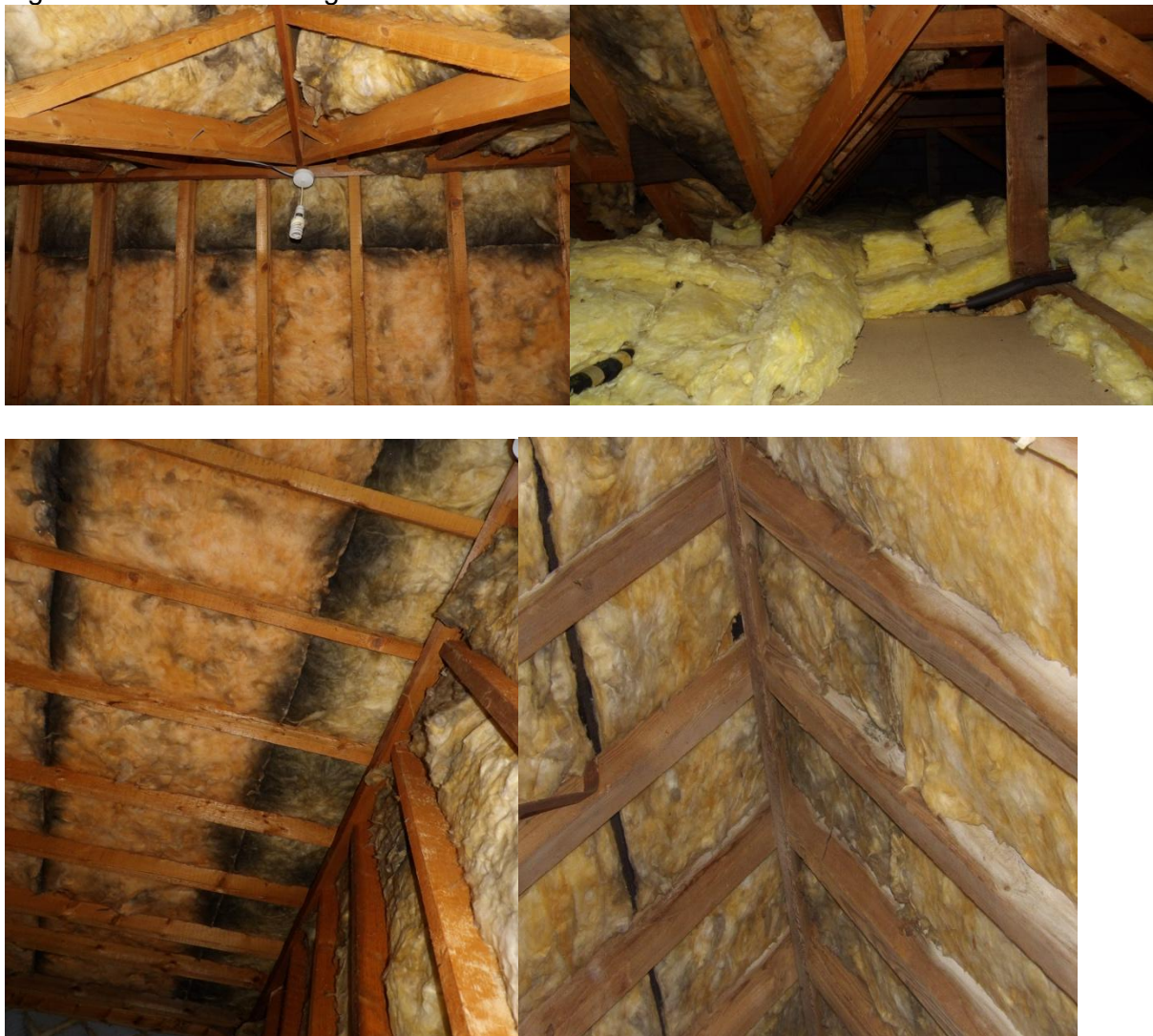
Figure 1/2/3. Main dwelling roof voids.
