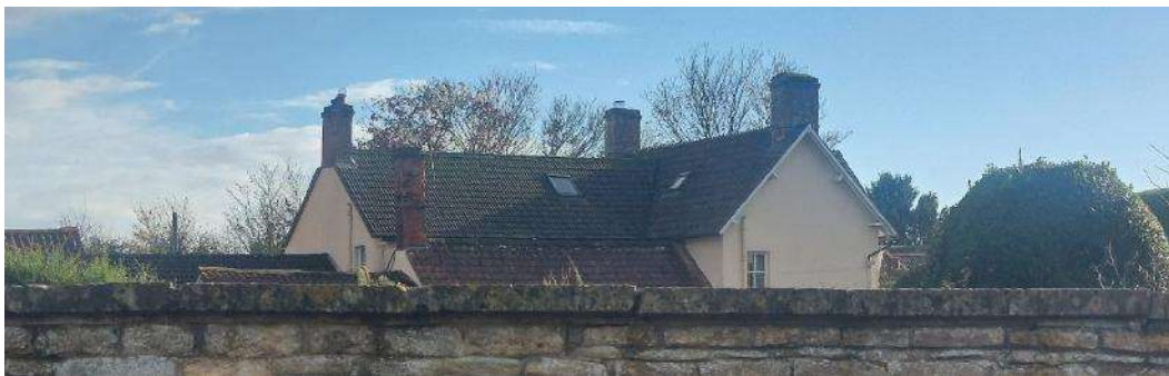
Figure 11 Rooflights to the rear roof slope of a house seen from Church Street.
