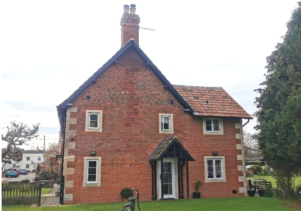
Figure 7 The north-west gable and modern rear extension.
