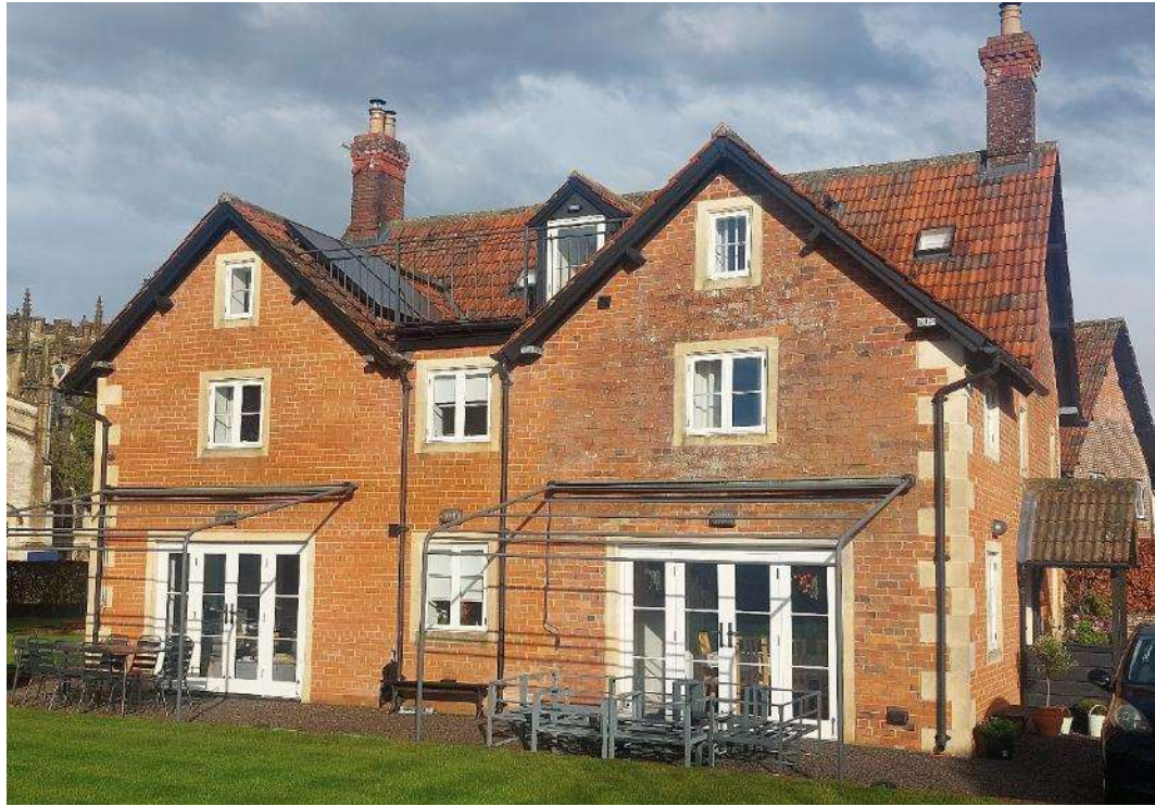
Figure 8 The solar panels to the inner roof slope of the modern extension as seen from the grounds of the house.
