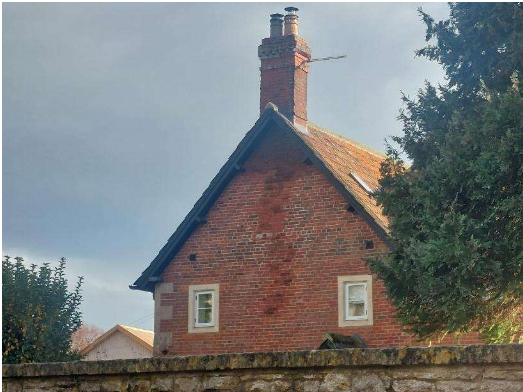
Figure 10 The limited view to the northern-most roof light from Church Street.
