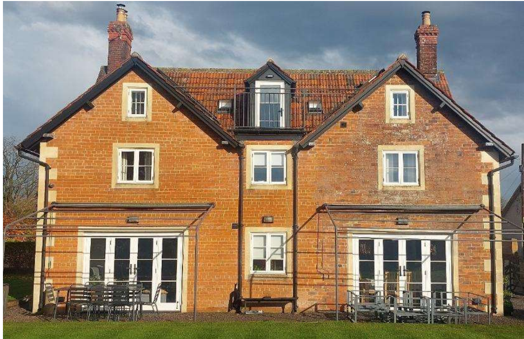
Figure 6 Rear elevation showing the historic wing to the right and the modern extension to the left.
