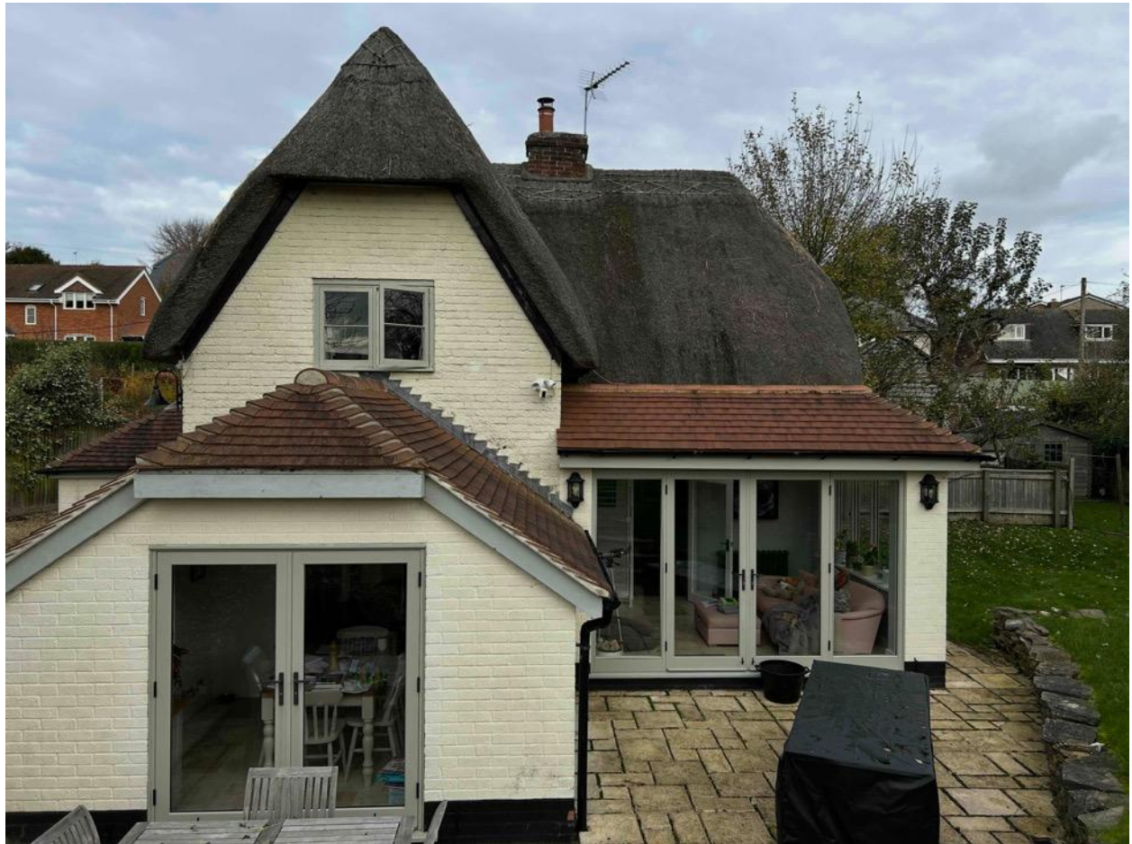
Rear Elevation – Chimney
