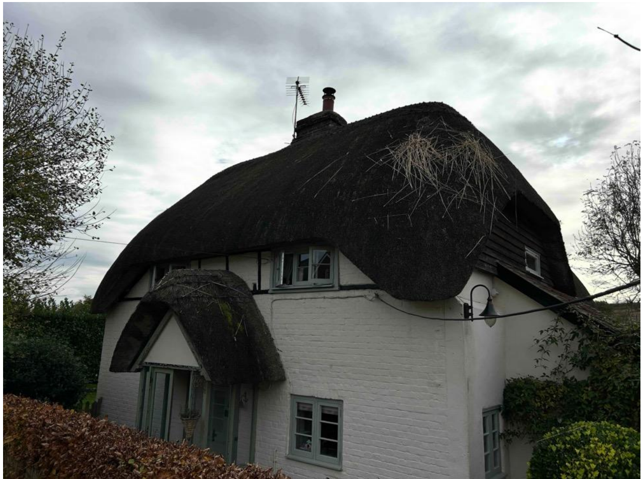
Front Elevation – Chimney
