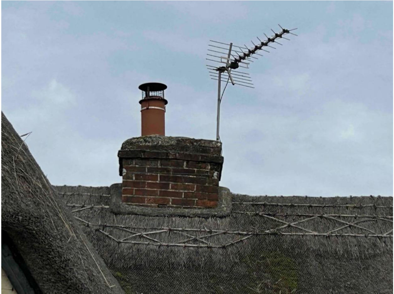
Close up – Chimney
