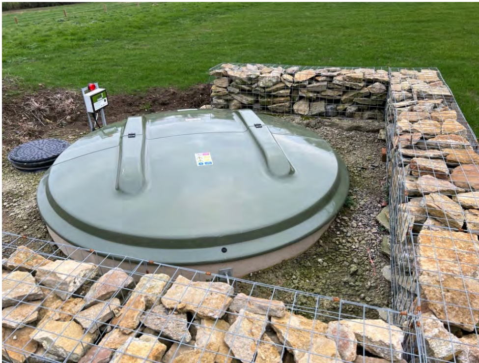
Klargester Biodisc - following installation
