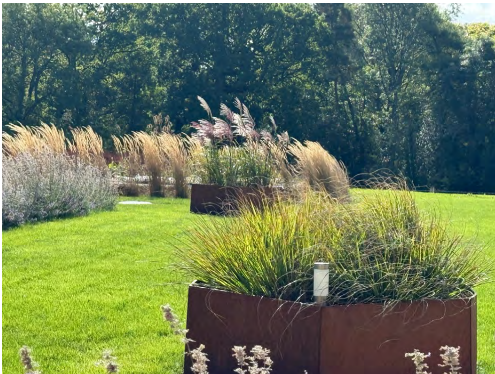
Views to the South - Klargester Biodisc screened by ornamental grasses
