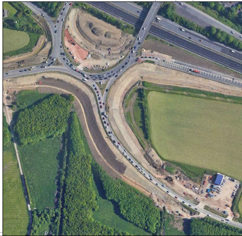
NORTH SOUTH AERIAL VIEW
