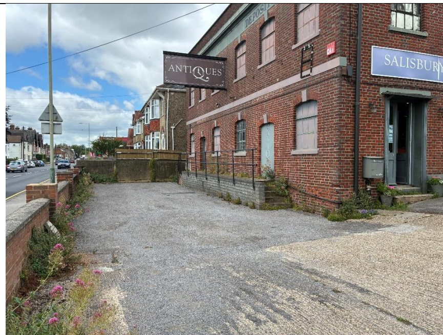
Plate 6: The open ground at the front of the existing building is slightly lower than Canadian Avenue and Wilton Road.
