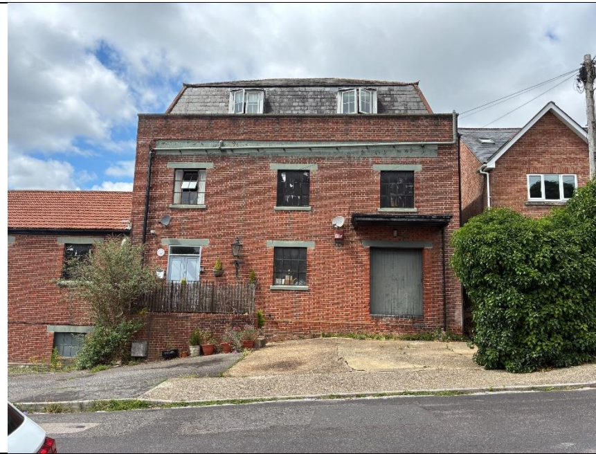
Plate 9: Facing the rear part of the PDA. This structure was built in 1926 and it has a basement and three floors above ground. The larger extension, which runs towards Wilton Road was built in 1928.
