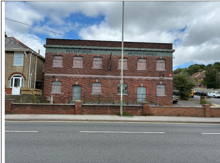
Plate 2: View towards the Salisbury Antiques Centre (PDA). We note the 'Pickfords Depositories' label on the building.
