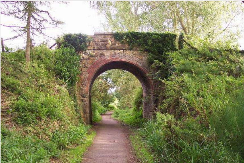
Above: The old railway bridge at the crossroads between Studley Hill and Stanley Lane. This pathway connects into Chippenham Town Centre.
