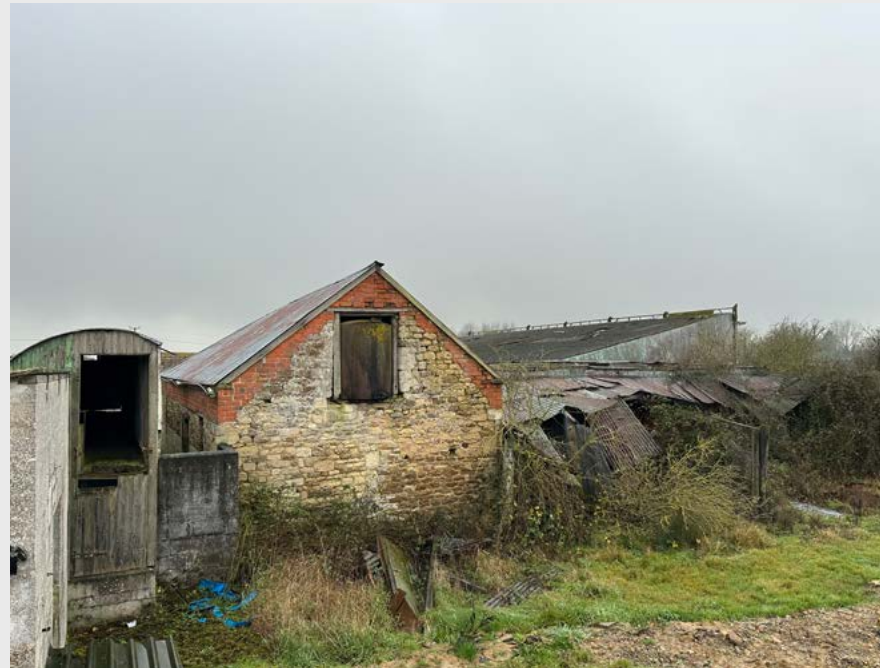
View of the front gable facing the road.
