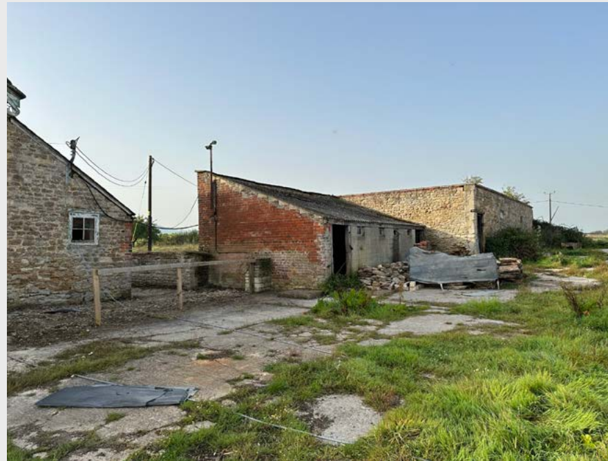
View from the yard: The brick wall of the cowshed can be seen here with the rear stone wall of the pig stys behind. The Cowshed has a mono pitched roof with breezeblock infill and door openings to the lower elevation.
