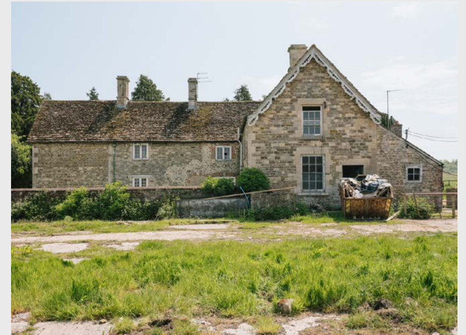
View across the courtyard towards the house. The barns are both visually and physically connected to the house and an important part of the setting. The historic relationship between the house and the farmyard is clearly visible.
