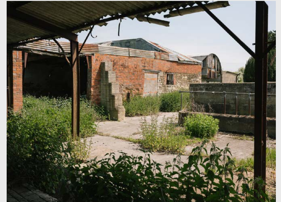
View from the large open sided barn adjacent to the granary. A buttress has been installed to prevent movement of the wall.
