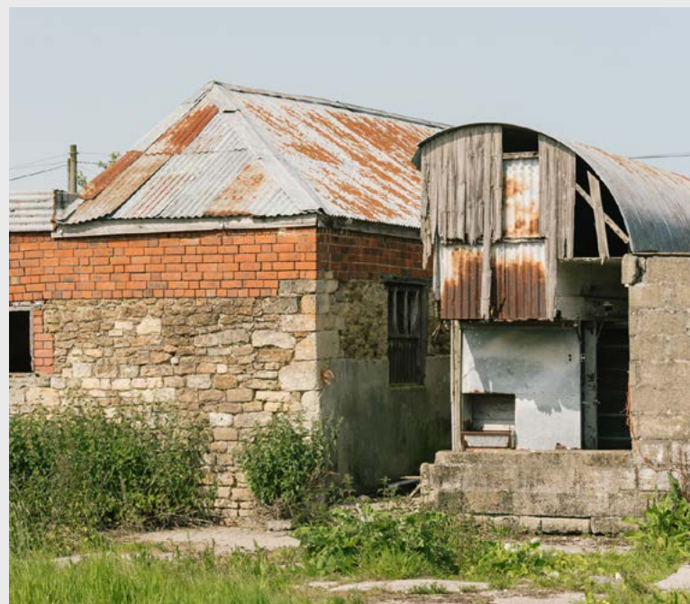
Stone corner detailing of the granary walls. Redundant curved roof milking parlour which is to be demolished.
