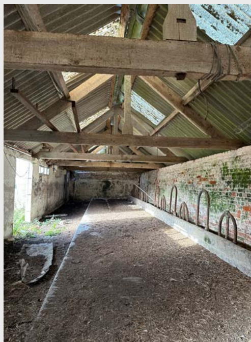
Good quality timber roof trusses which remain in good condition. The asbestos roof linings will be replaced and the walls locally repaired.
