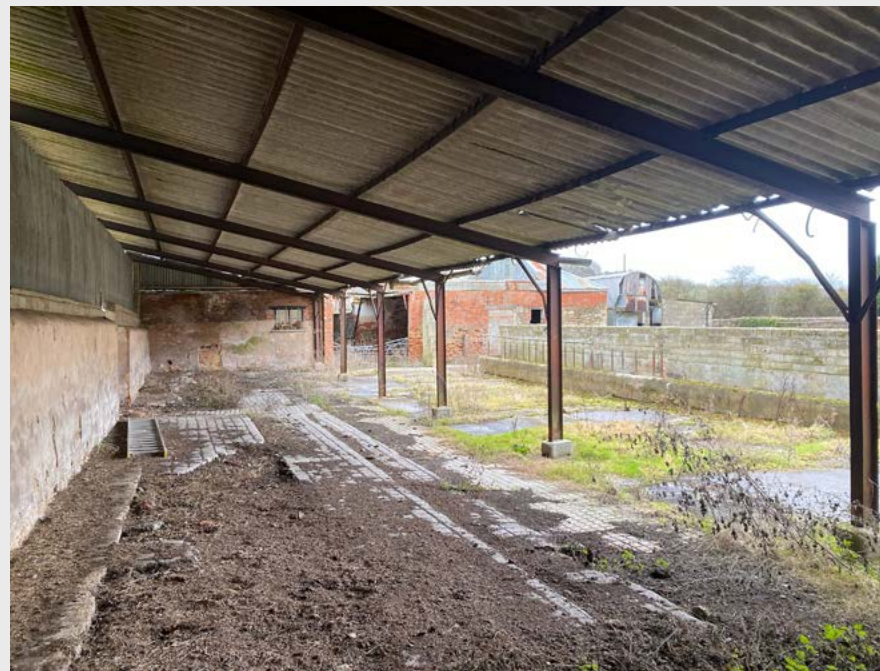
View looking out to yard with tall, thick stone wall to the left.
