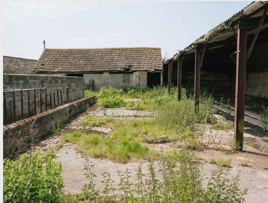
View of the barn to the right with the large mono-pitched roof and exposed steel frame. To the left is the large concrete cattle feeder which blocks views across the courtyard and will be removed.
