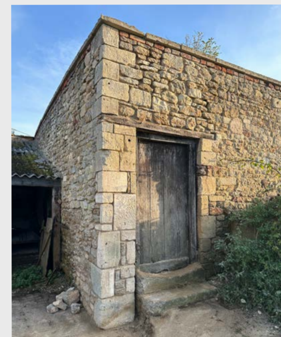
The brick & stone walls are well built and remain in good condition. The stone style suggests there might previously have been a larger stone structure here which was converted to the smaller pig stys.
