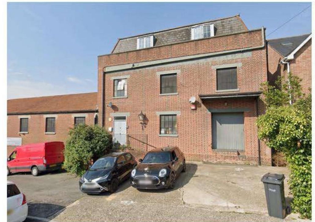
View of existing buildings Penthouse entrance
