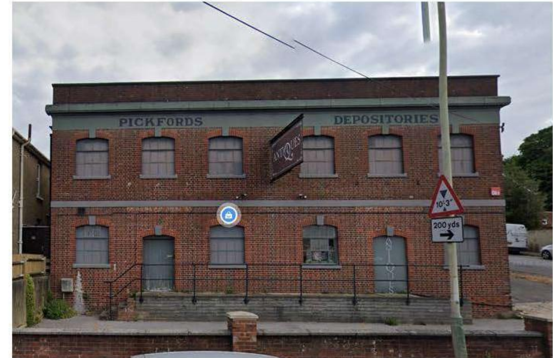
View of existing building south/front elevation
