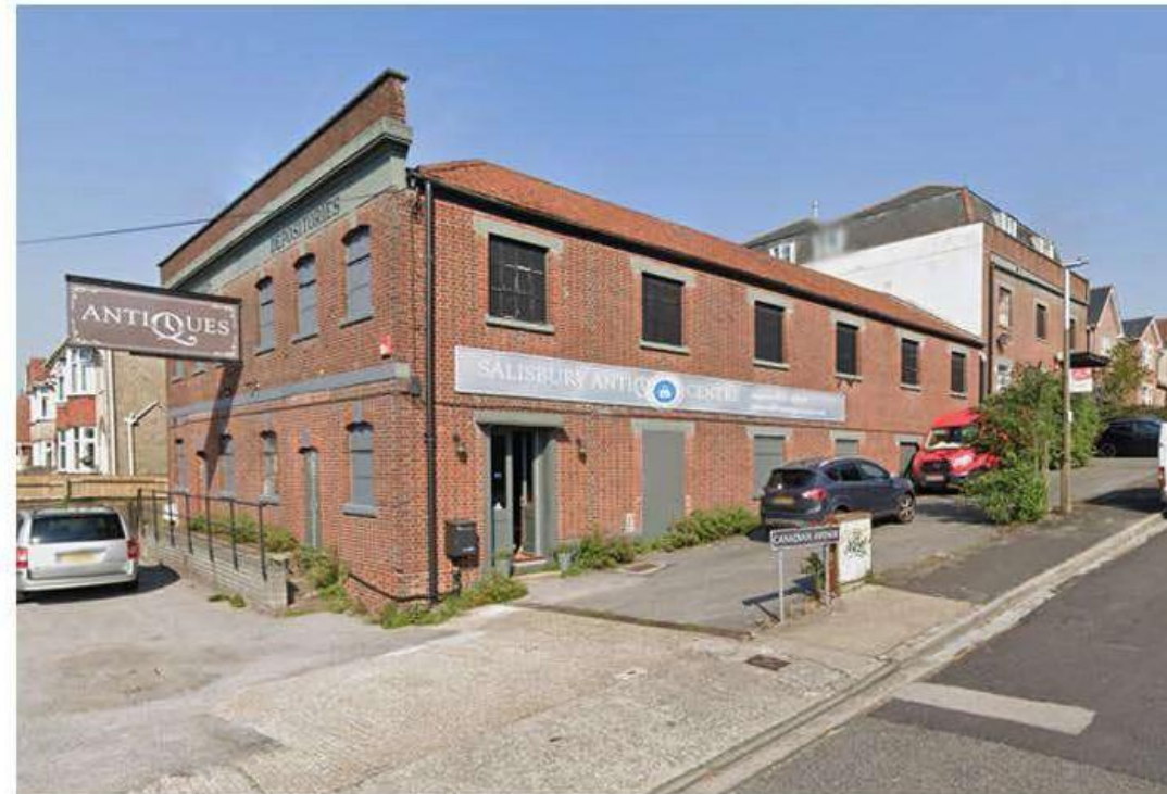
View of existing building south and east elevations
