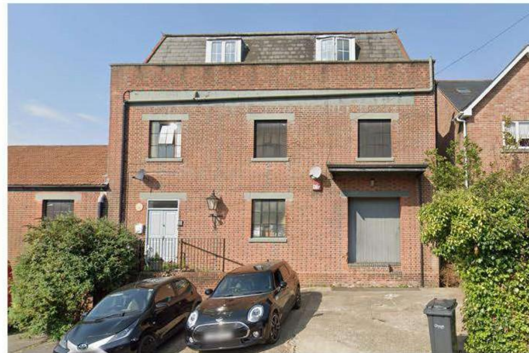
View of buildings east elevation and Penthouse entrance
