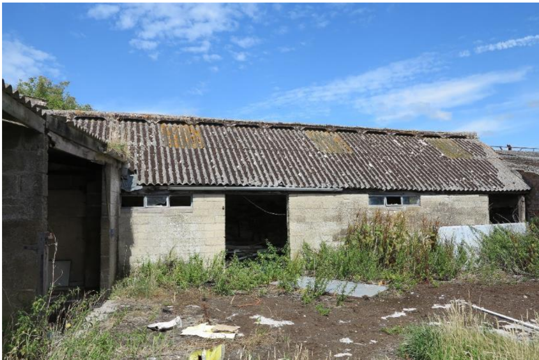
Plate 44. Structure 4 was historically a shelter shed, open onto the south-western foldyard on its southern elevation; however, this has been infilled in blockwork
