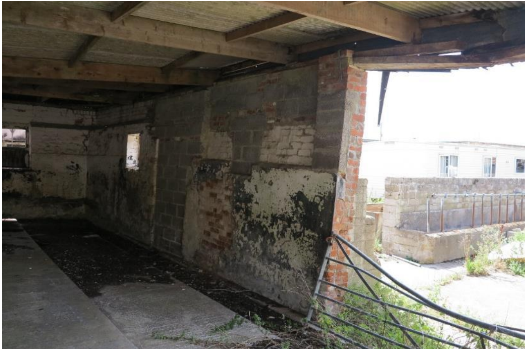
Plate 31. Parts of the southern wall of structure 1 have been rebuilt in blockwork
