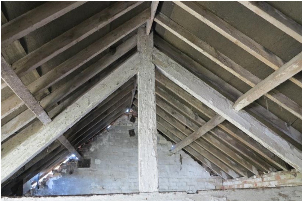
Plate 40. King-post truss and later replacement purlins and rafters in structure 3
