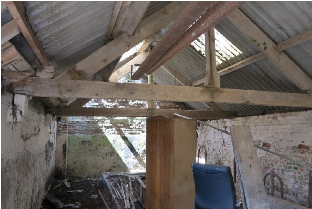
Plate 47. King-post truss in structure 4
