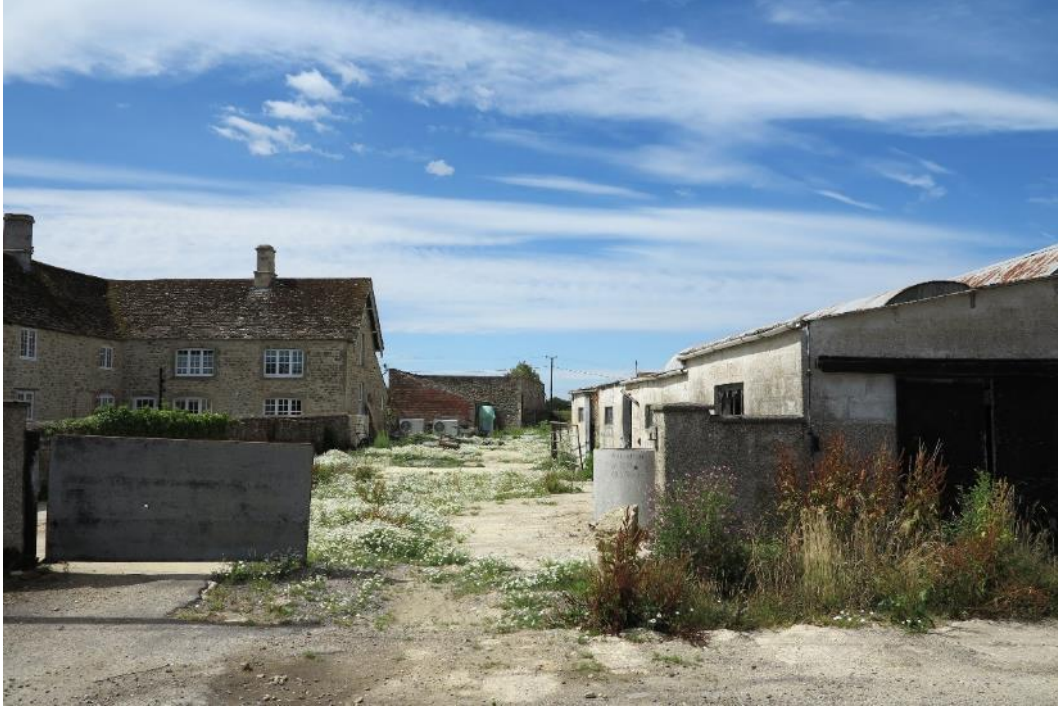
Plate 19. Looking into the yard from the road; from this angle any views of the traditional farm buildings on the northern side are curtailed by the modern structure 9
