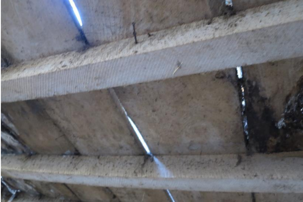
Plate 25. While historic boards have been reused, the first-floor structure in structure 1 is constructed with circular-sawn joists
