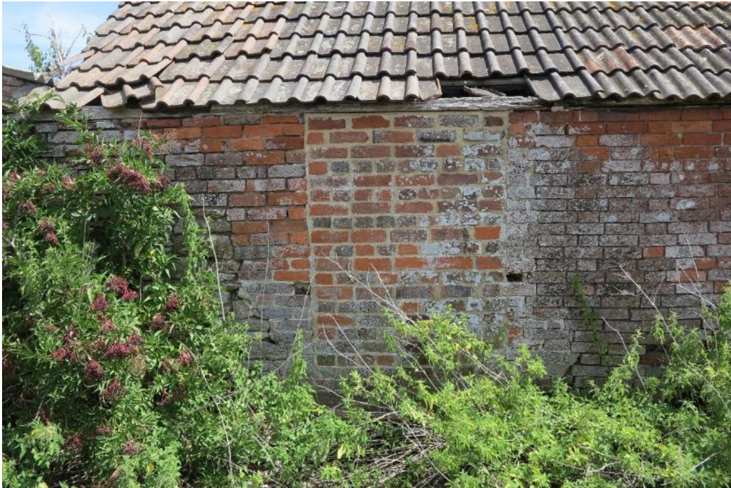
Plate 37. A historic doorway on the south-western elevation of structure 3 has been infilled
