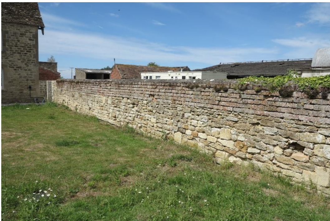
Plate 16. The tall boundary wall between the house and yard; note, the only opening in this wall is where it has been rebuilt at the western end
