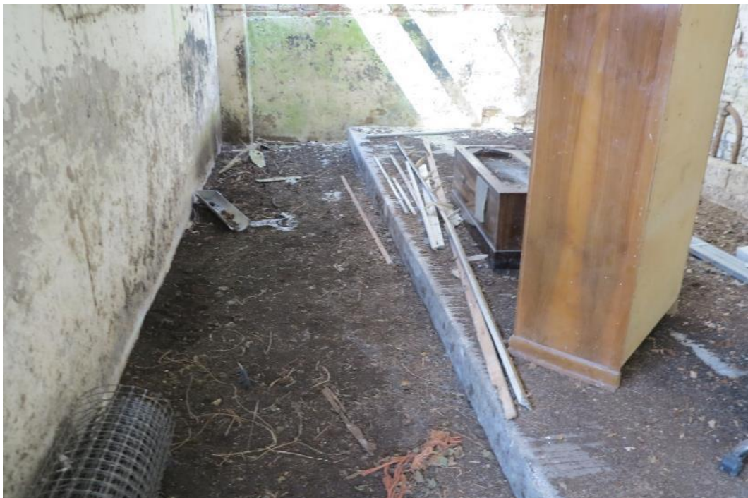
Plate 2. The lower element of the central wall within structure 2 relates to the rear wall of the earlier shelter shed in this location
