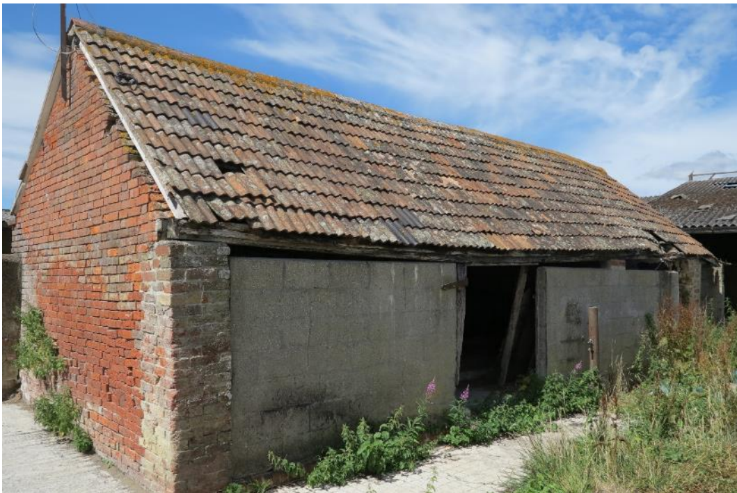
Plate 38. Structure 3 was historically a shelter shed, open onto the central foldyard on its north-eastern elevation; however, this has been infilled in blockwork
