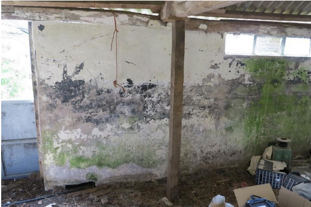
Plate 3. Structure 4; formerly open-fronted shelter sheds on the site have been infilled in blockwork
