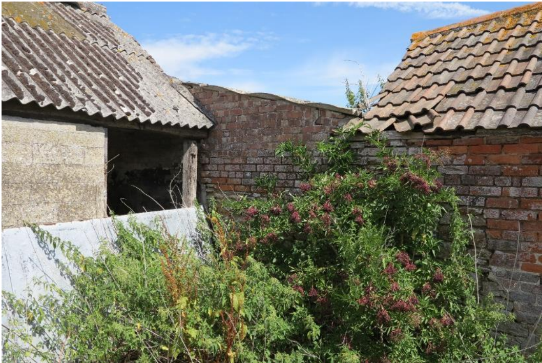
Plate 42. The WC structure at the north-western end of structure 3 incorporates parts of an earlier wall
