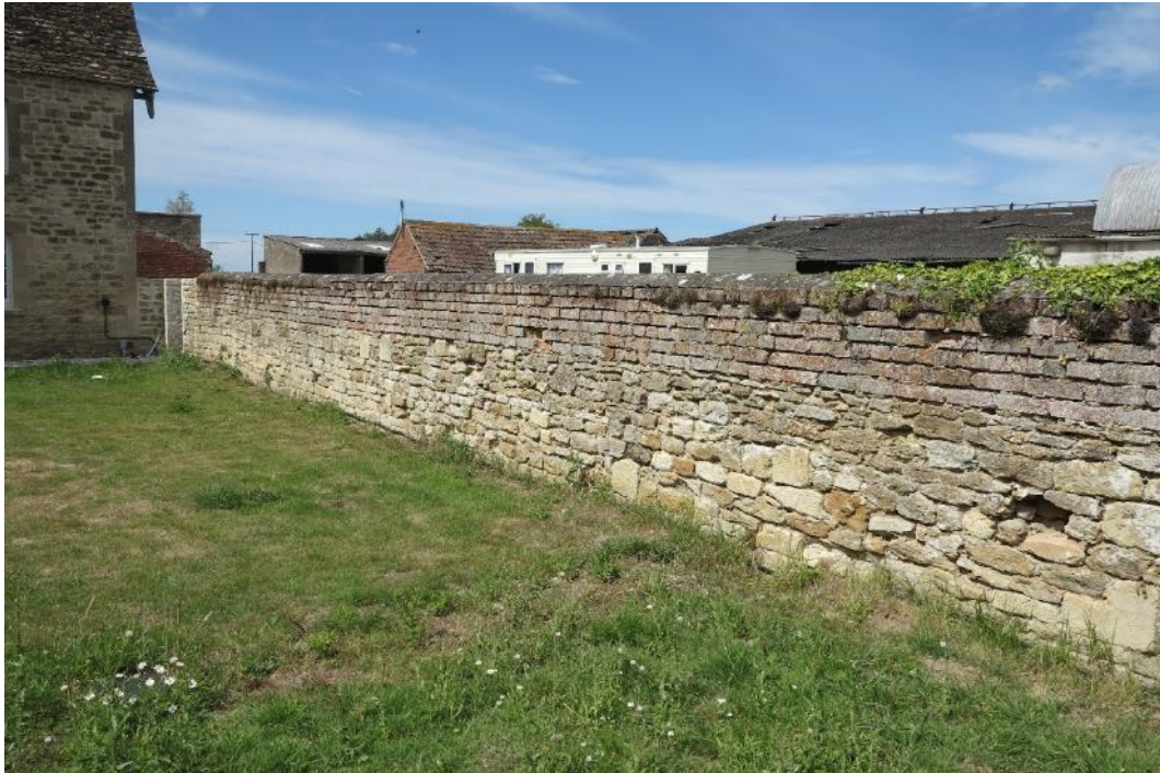
Plate 1. The boundary wall between the residential curtilage of the farmhouse and the agricultural yard
