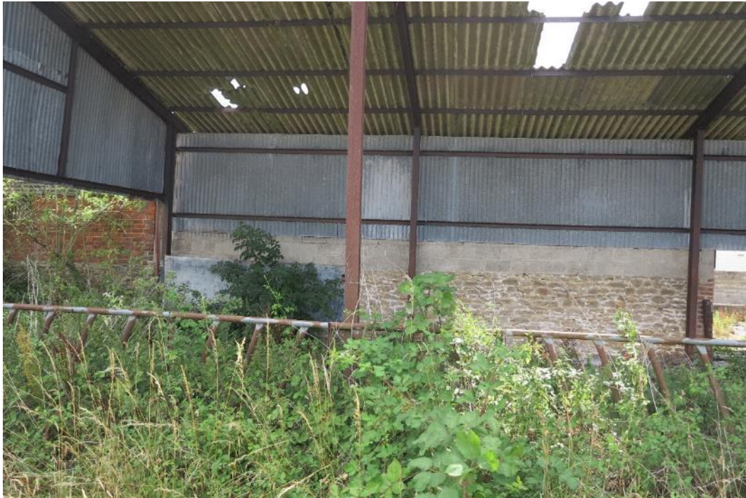
Plate 33. The lower element of the central wall within structure 2 relates to the rear wall of the earlier shelter shed in this location
