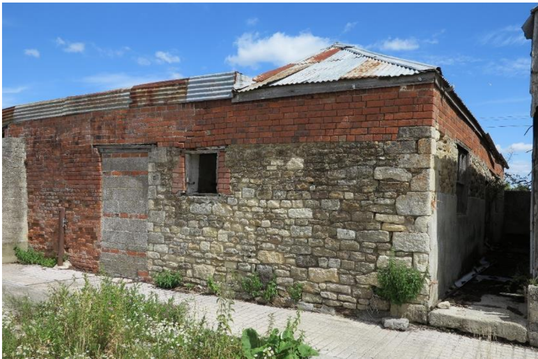
Plate 22. The south-western elevation of structure 1, where the earlier, stone-built stable has been incorporated into the later range
