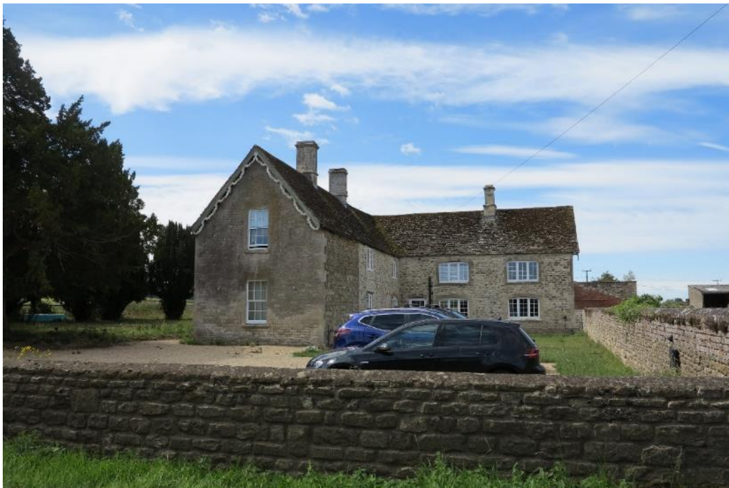
Plate 14. The house from the road, looking over its roadside boundary wall; note the taller boundary wall to the agricultural yard on the right
