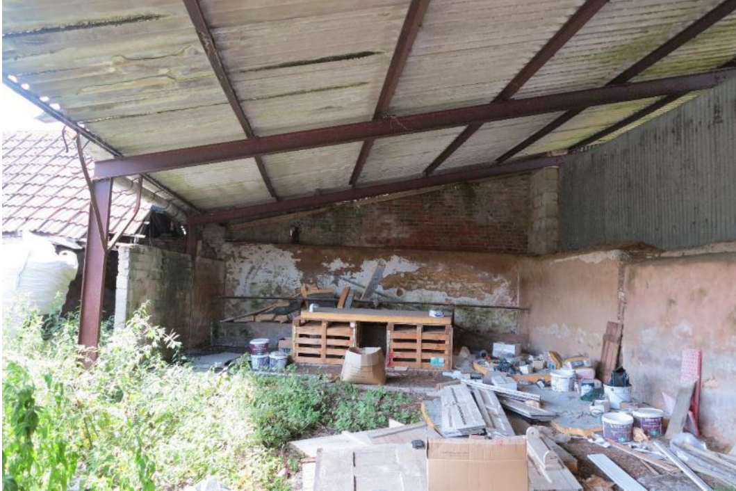
Plate 35. Structure 3 from the south
