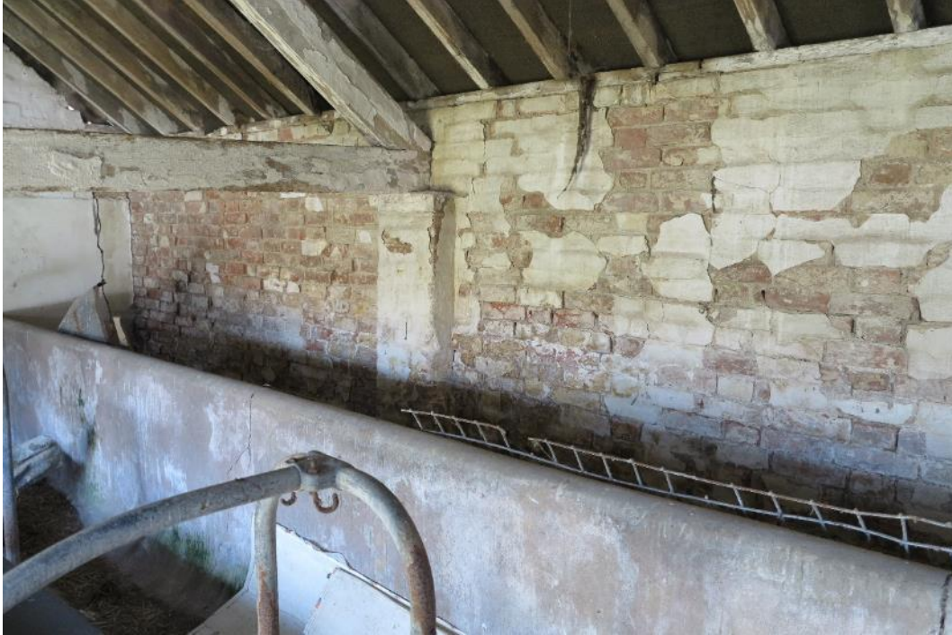
Plate 41. Concrete troughs in structure 3
