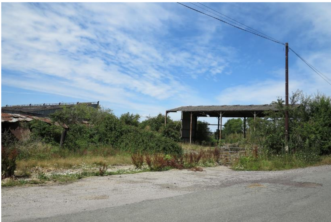
Plate 34. Structure 2 is a modern, open-fronted, metal shed
