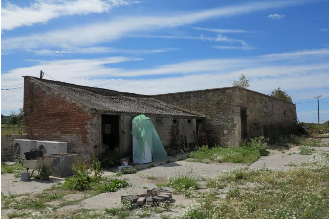
Plate 51. Structure 6 was historically a shelter shed, open onto the south-western foldyard on its northern elevation; however, this has been infilled in blockwork
