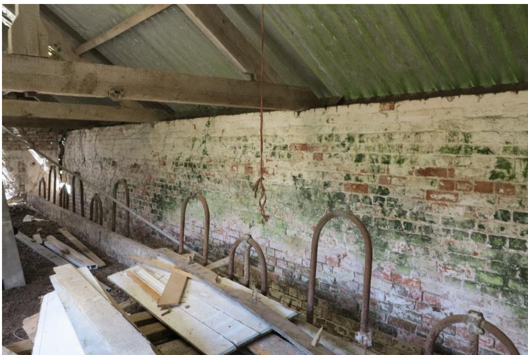
Plate 48. Concrete troughs in structure 4
