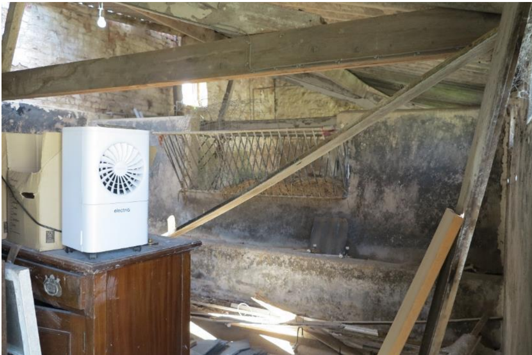
Plate 52. Modern stalls have been inserted within structure 6
