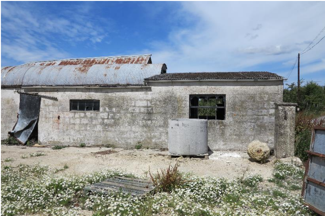
Plate 54. The milking parlour (structure 9)
