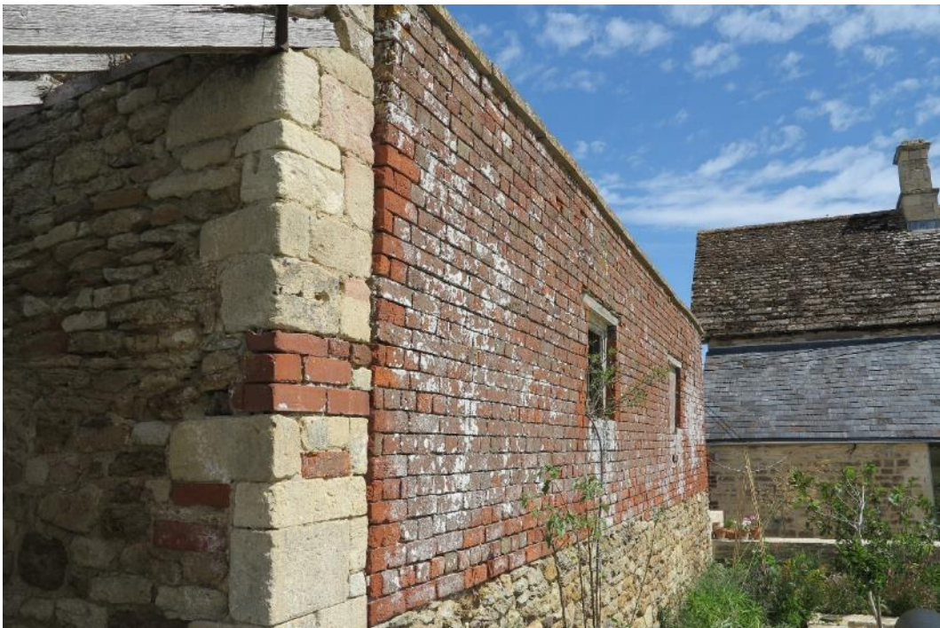
Plate 50. The rear wall of structure 6 from the farmhouse garden
