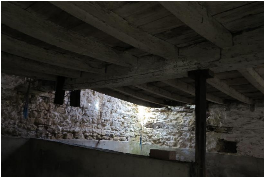
Plate 24. The surviving first-floor structure at the northern end of structure 1
