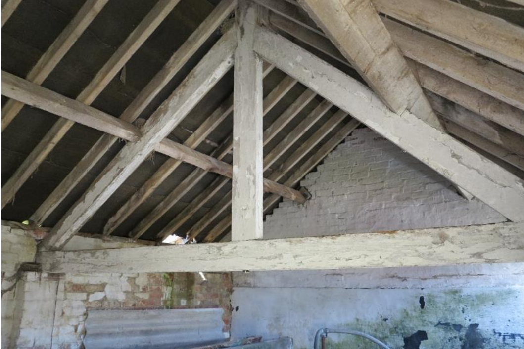
Plate 39. King-post truss in structure 3
