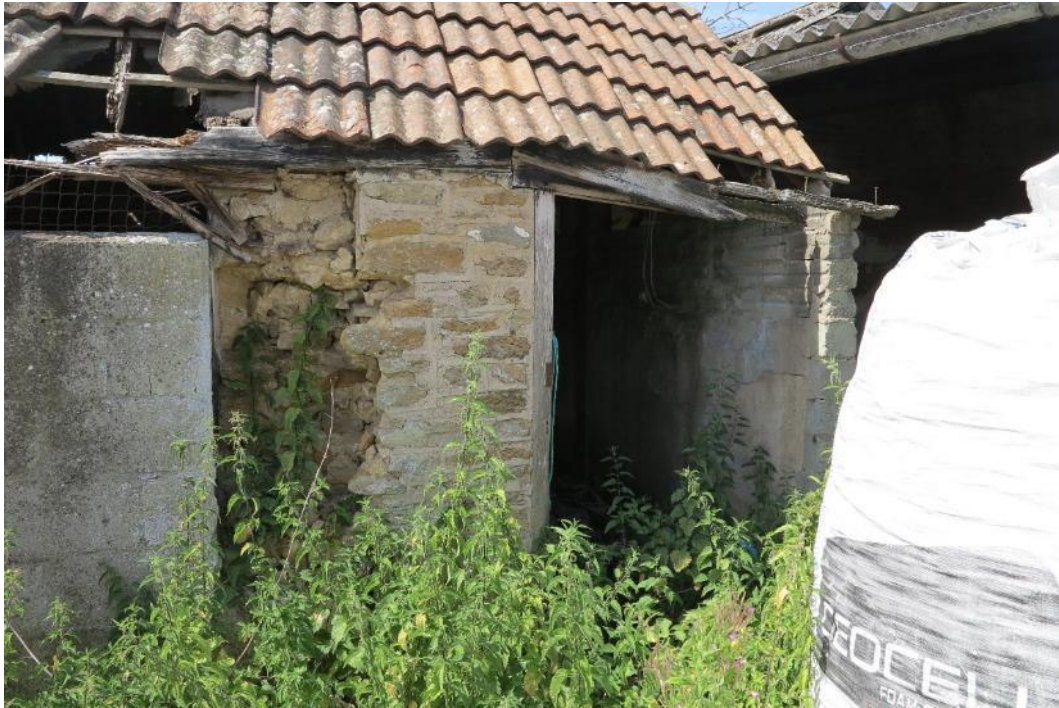
Plate 43. The WC structure at the north-western end of structure 3
