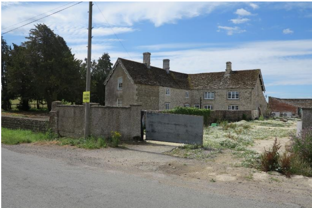
Plate 10. Looking from the road across the yard entrance onto the farmhouse
