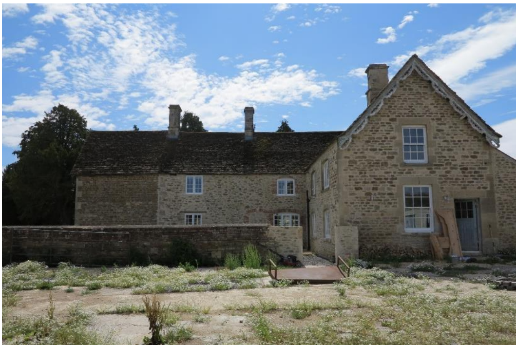
Plate 4. The rear of Pound Farmhouse showing the boundary wall between the house and yard; the area of wall behind the rear range has been demolished and its junction with the surviving stretch of wall rebuilt since 2001
