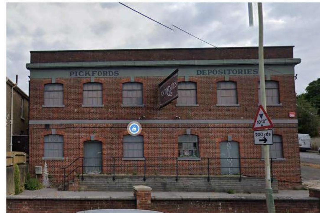
View of existing building south/front elevation
