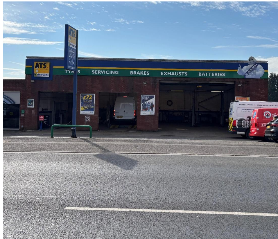
View of existing commercial property to the immediate south
