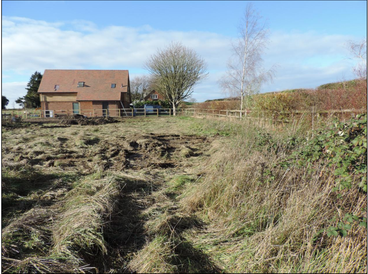
Photo 2: West facing view of site showing new build development as part of 21/00584/F.
