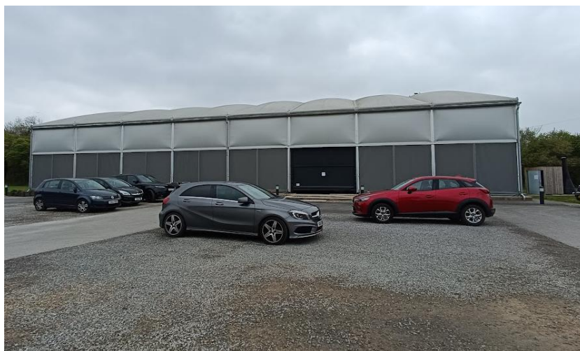
Figure 2: Existing Padel Courts
