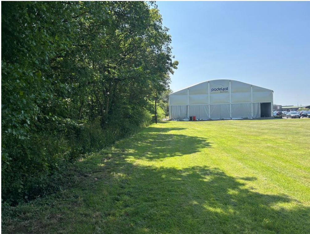
Photograph 2. B1; padel courts
