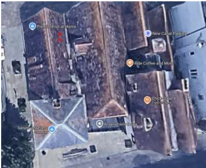
Picture 5a – Roof extractors (red)
