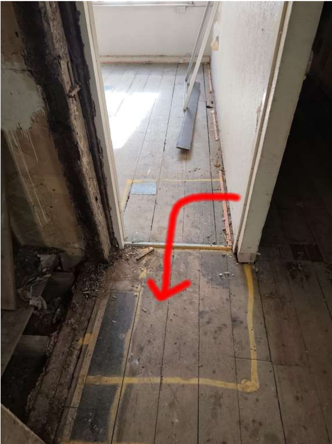
Picture 8b. New entrance door for Flat 3
