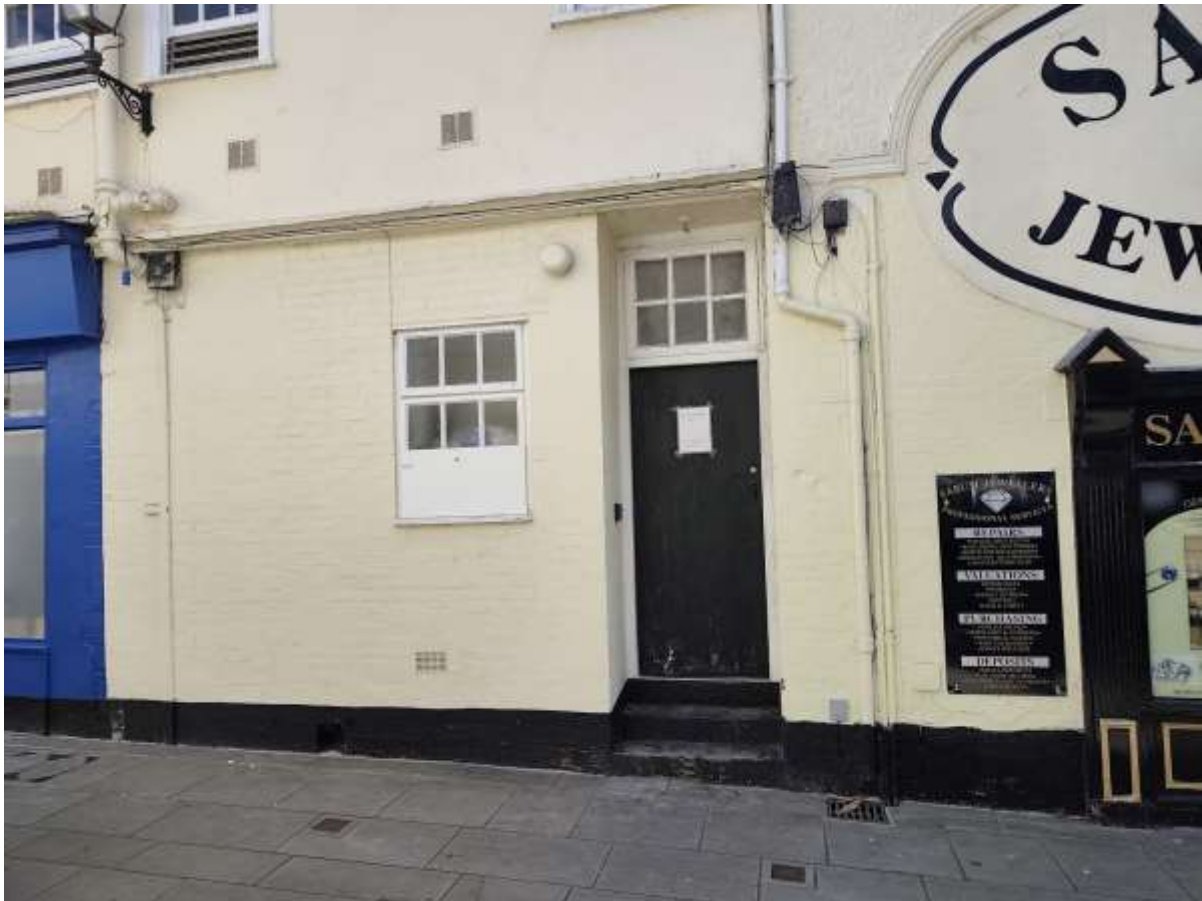
Picture 6a – Residential entrance (existing)
