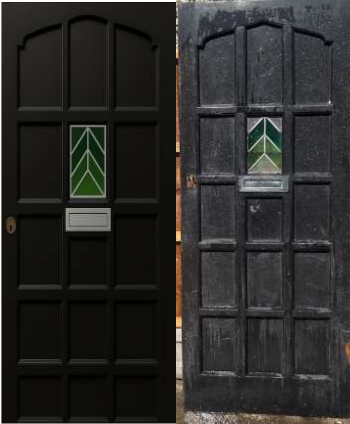
Picture 6c – Residential door details (restored, unrestored)
