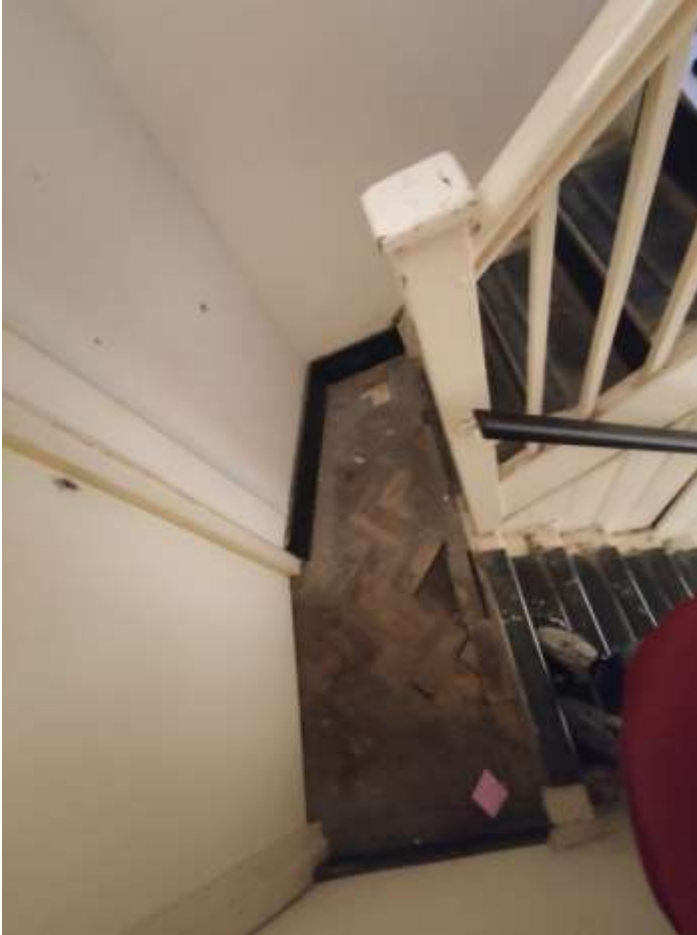
Picture 1b – Communal staircase current reduced half-landing
