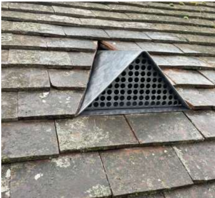
Picture 5b – Lead Roof Vent proposed
