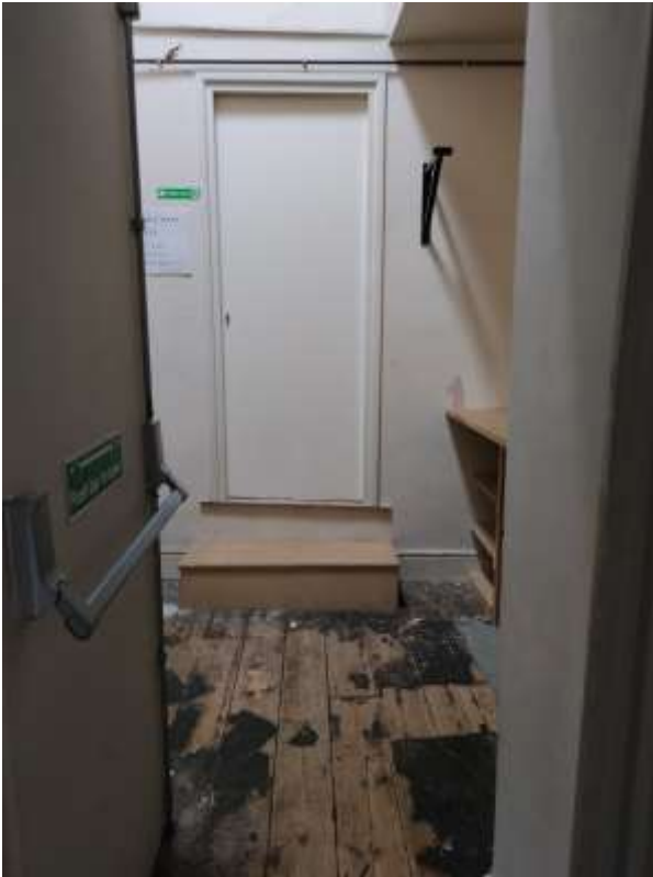
Picture 2 – 9 Fish Row emergency exit door to be removed and opening sealed
