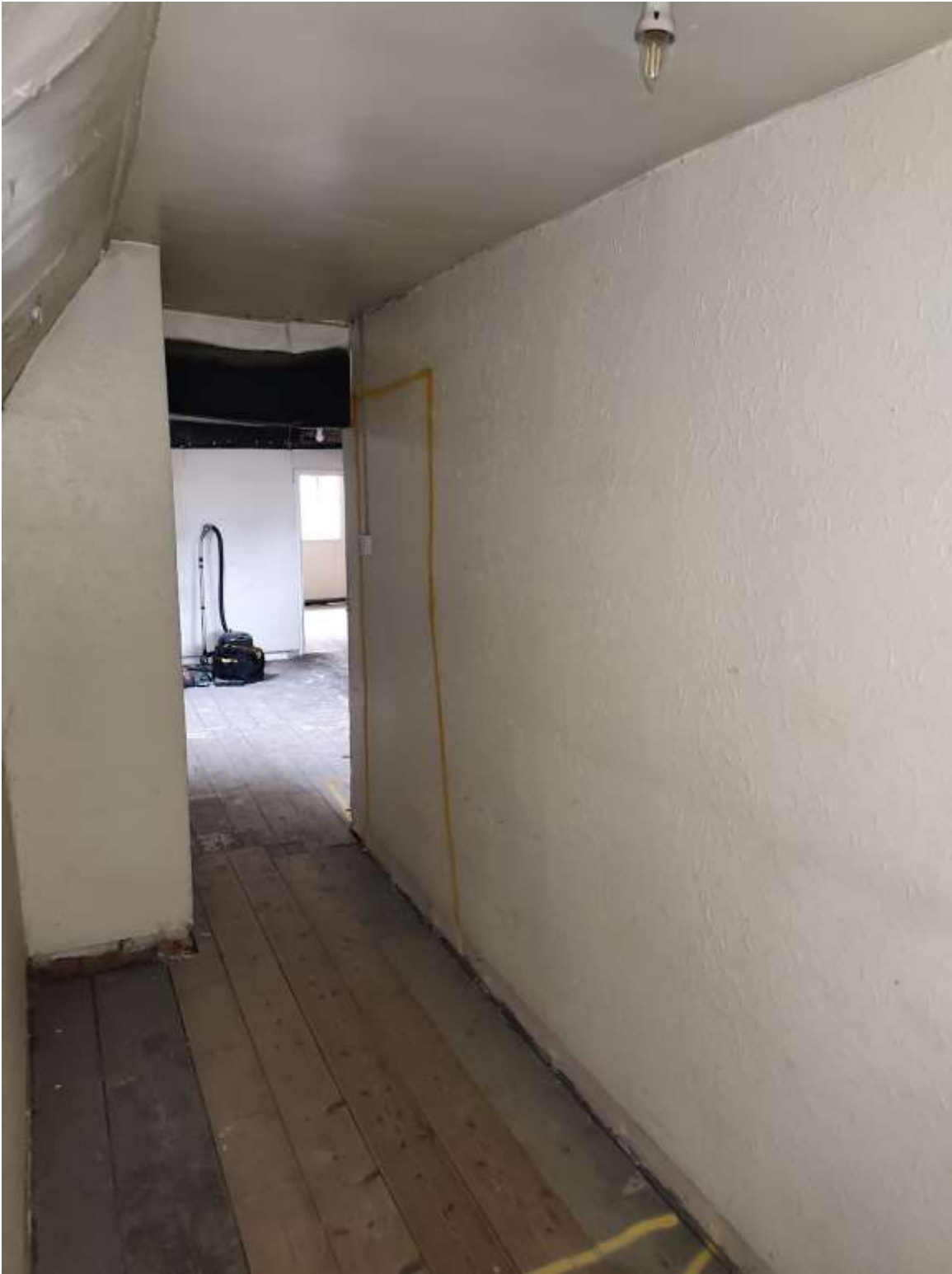
Picture 8a. New entrance door for Flat 3
