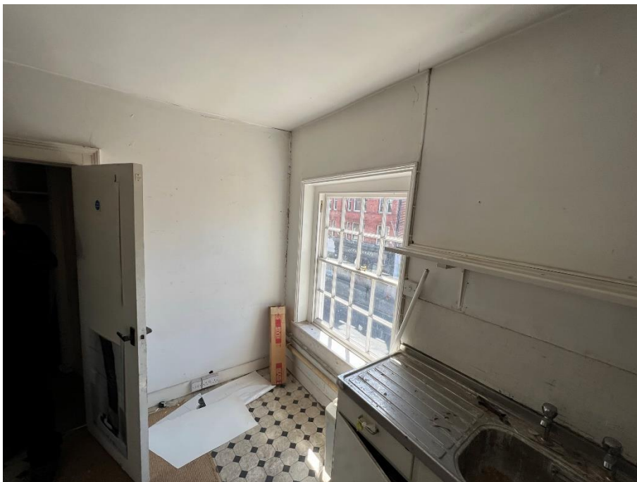
Photograph 18 7 and 9 Fish Row, Salisbury SP1 1EX Room 5 – Facing East – in reasonably good condition
