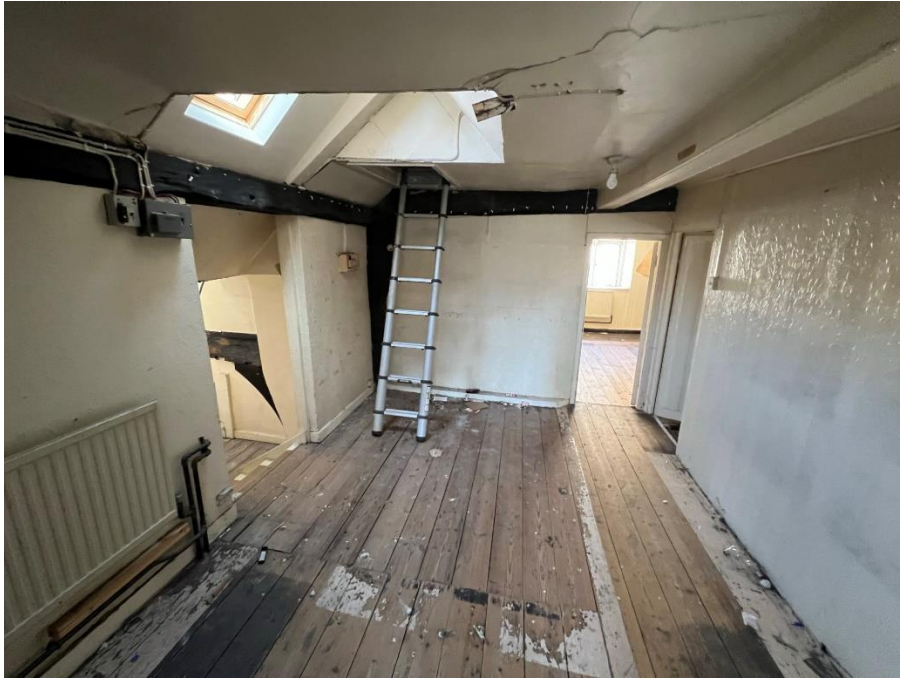
Photograph 15 7 and 9 Fish Row, Salisbury SP1 1EX Communal Area – Facing North – in reasonably good condition
