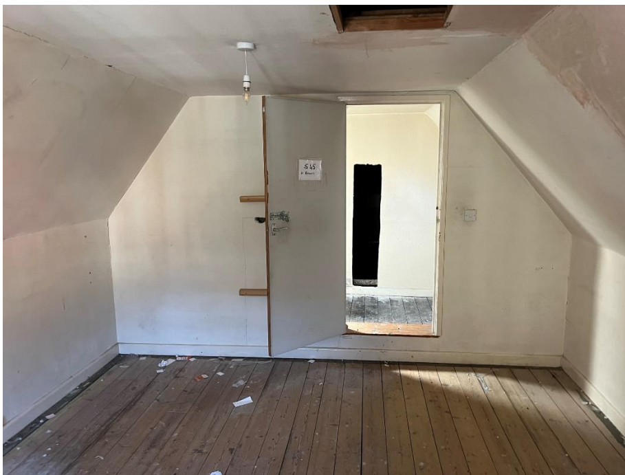
Photograph 06 7 and 9 Fish Row, Salisbury SP1 1EX Room 1 – Facing South – in good condition
