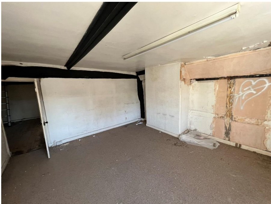
Photograph 14 7 and 9 Fish Row, Salisbury SP1 1EX Room 4 – Facing North – in reasonably good condition
