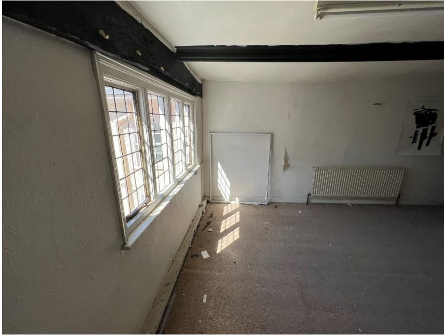
Photograph 13 7 and 9 Fish Row, Salisbury SP1 1EX Room 4 – Facing West – in reasonably good condition
