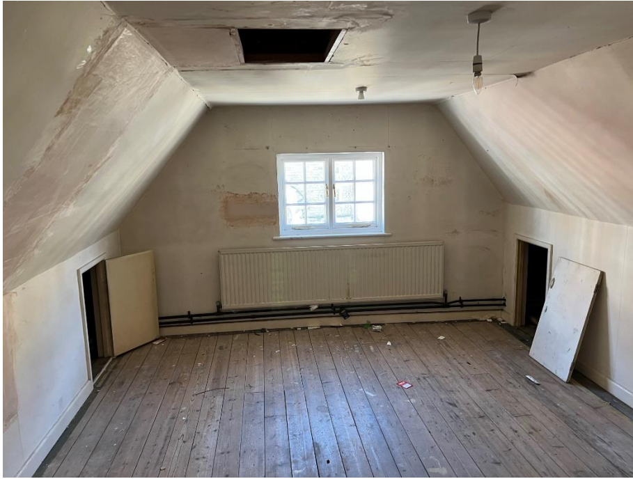
Photograph 05 7 and 9 Fish Row, Salisbury SP1 1EX Room 1 – Facing North – in good condition
