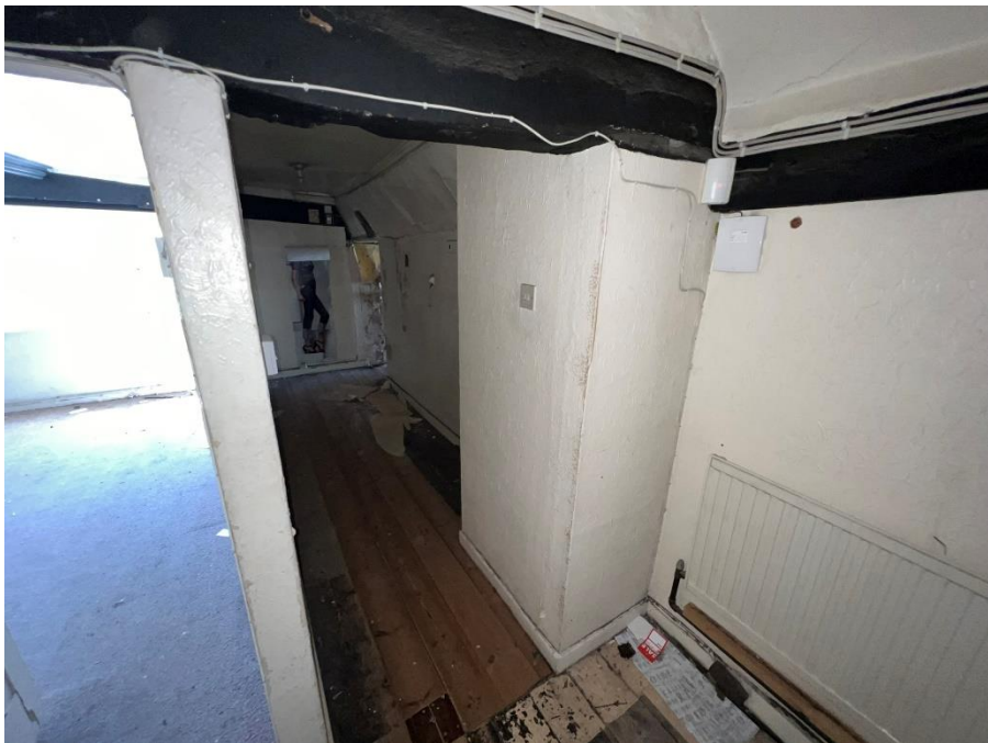
Photograph 16 7 and 9 Fish Row, Salisbury SP1 1EX Communal Area – Facing South – in reasonably good condition
