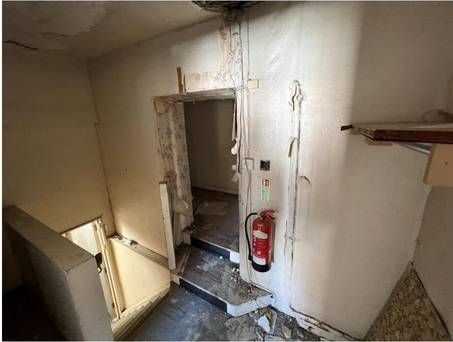
Photograph 17 7 and 9 Fish Row, Salisbury SP1 1EX Communal Area – Facing East – in reasonably good condition
