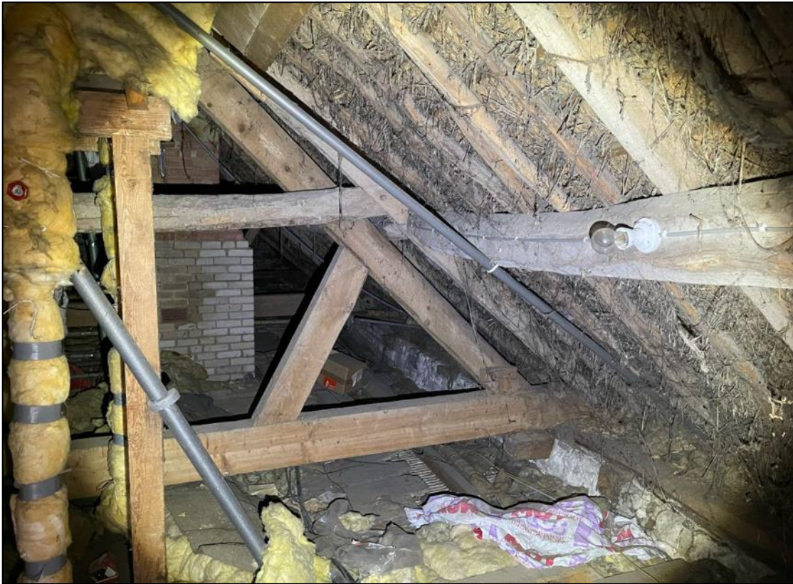
Manor Barn roof structure showing replaced main truss and mid C20 chimney.
