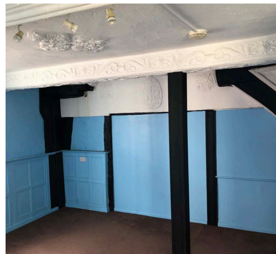
figure 16: First floor 17th century ornate plasterwork to beams and ceiling
