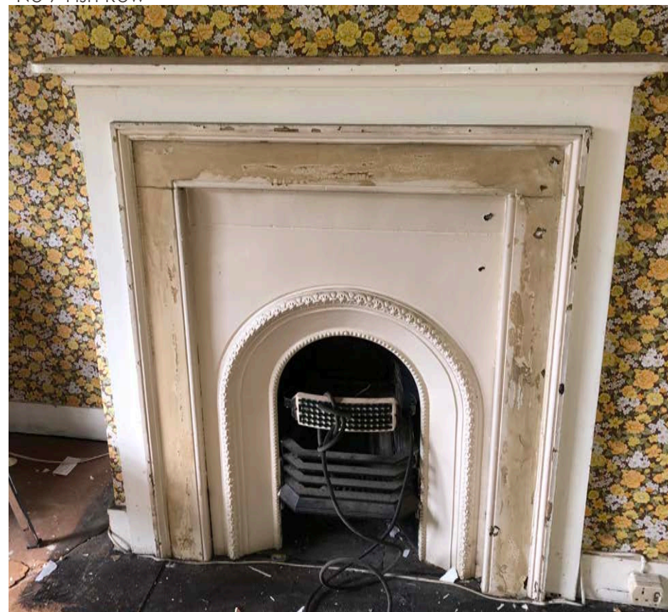
figure 17: early 19th century fireplace to second floor extension to rear of No 9 Fish Row
