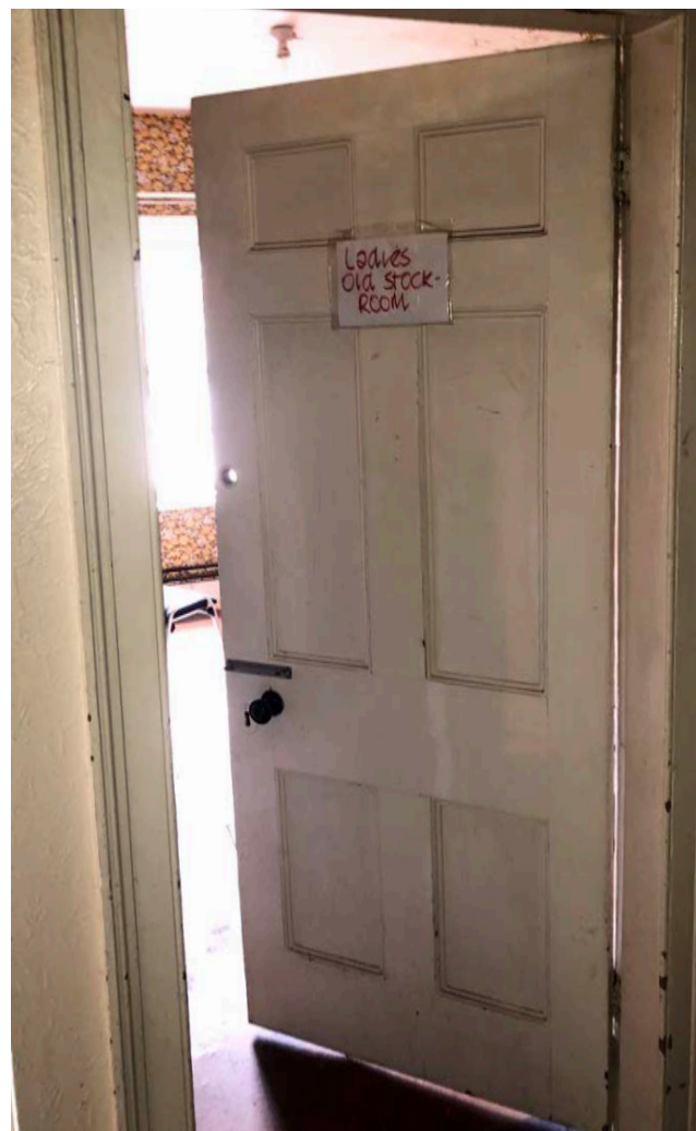
figure 25: possibly early 19th century 6 panel door D-16 is proposed to be upgraded for 30 min fire protection and remain in situ.
