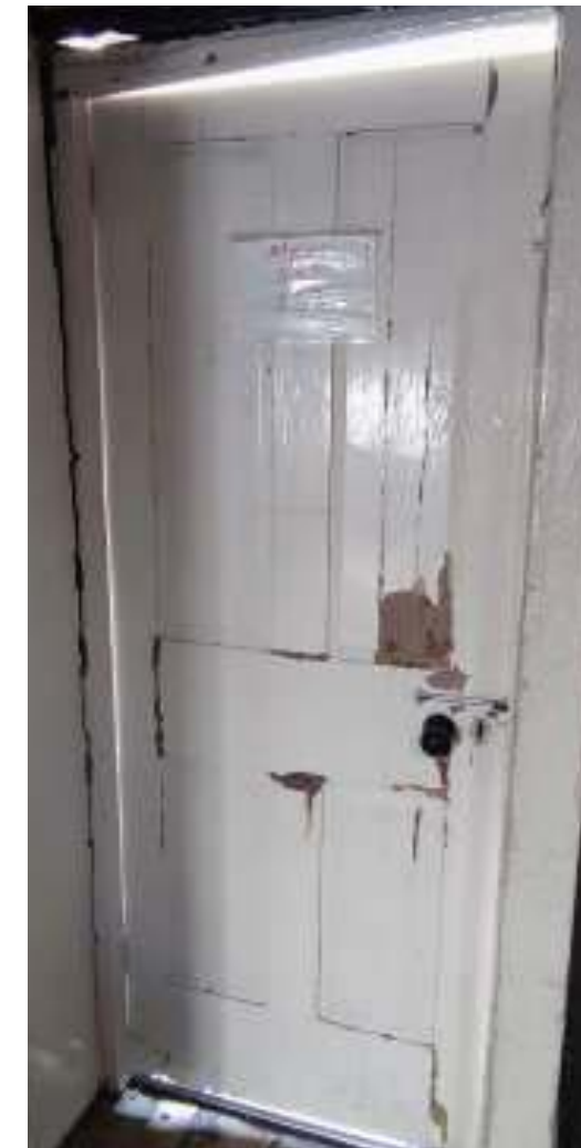
figure 28: D-27 appears to be a mid to late 19th century door. It will be salvaged, repaired and re-purposed.
