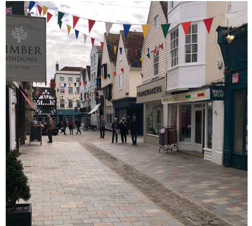
figure 23: No 7-9 Fish Row in the centre looking east and forming part of an important collection of historic buildings in a prime frontage identified in the local plan
