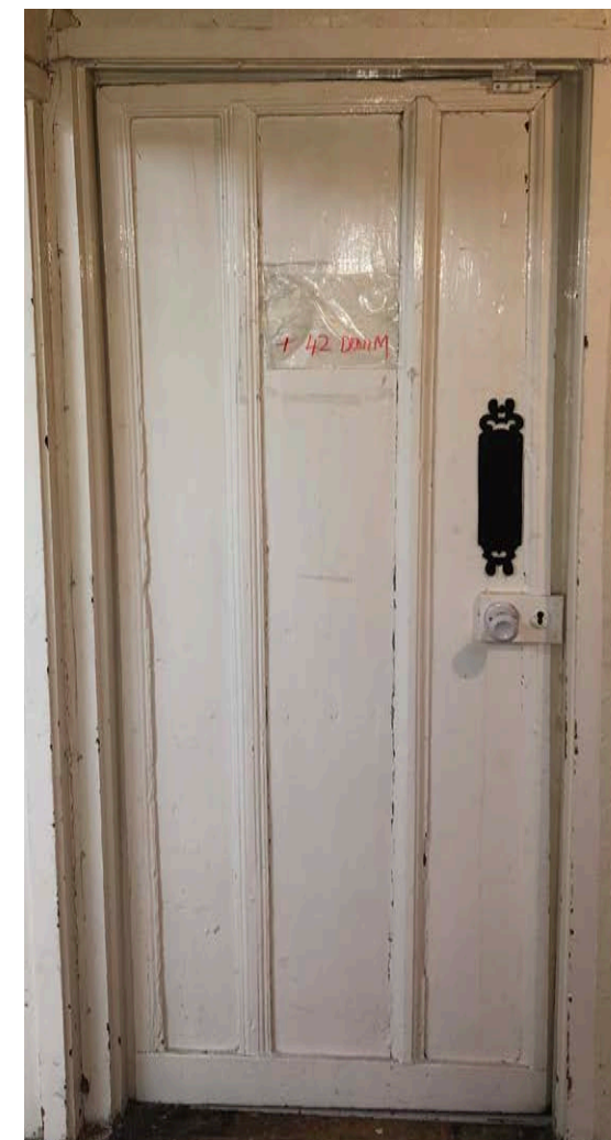
figure 27: D-20 appears to be a 16th or 17th century reused door. It will be salvaged, repaired and re-purposed with its ironmongery.
