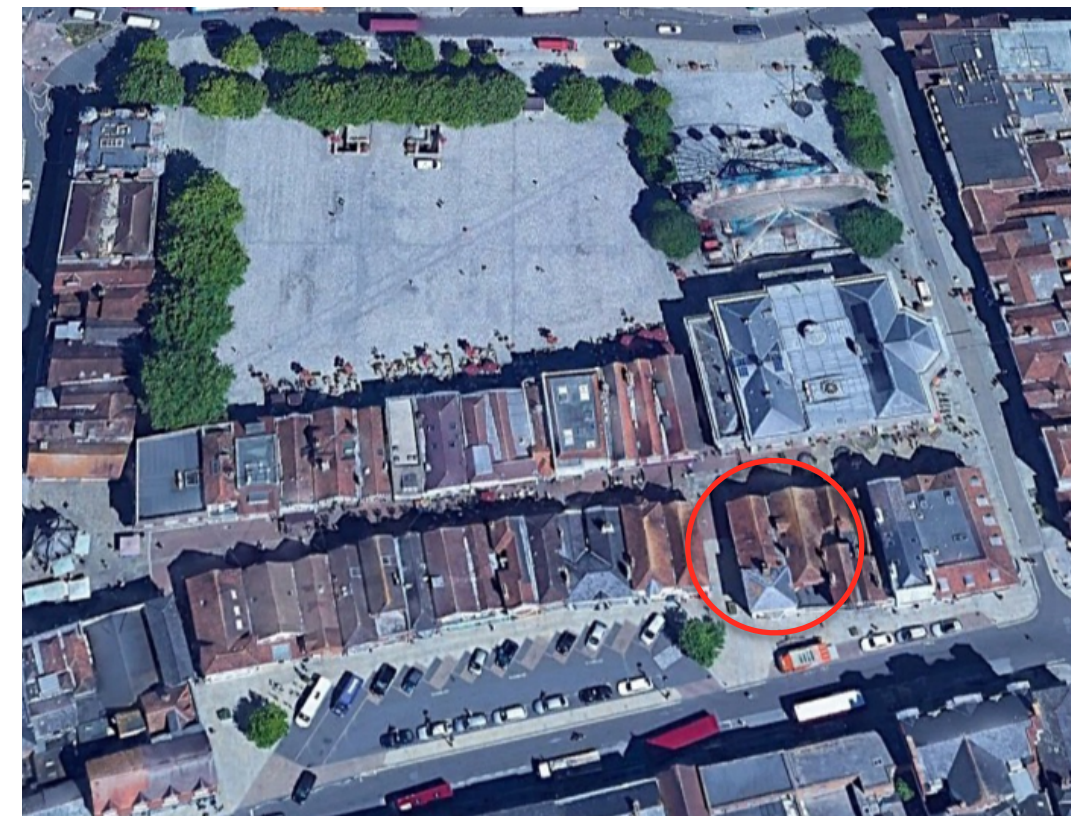
figure 9: 7 and 9 Fish row ringed. The 19th century extension to 9 Fish Row clearly identified with the hipped slate roof.
