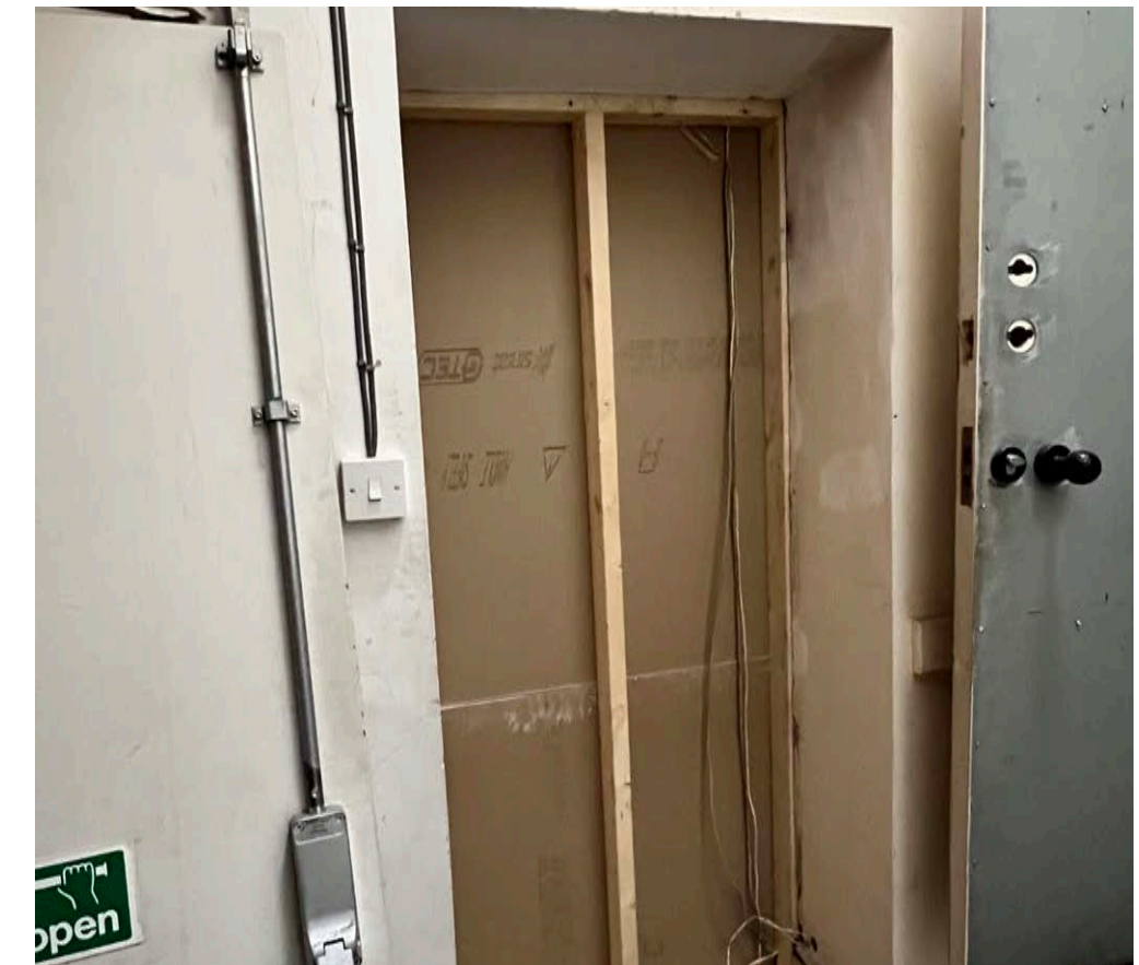
figure 32: 7 Fish Row blocked access from first floor to be re-opened with a traditional door and modern doors also removed.
