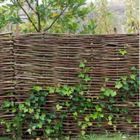
ILLUSTRATIVE EXAMPLE OF WILLOW HURDLE FENCING Scale N.T.S
