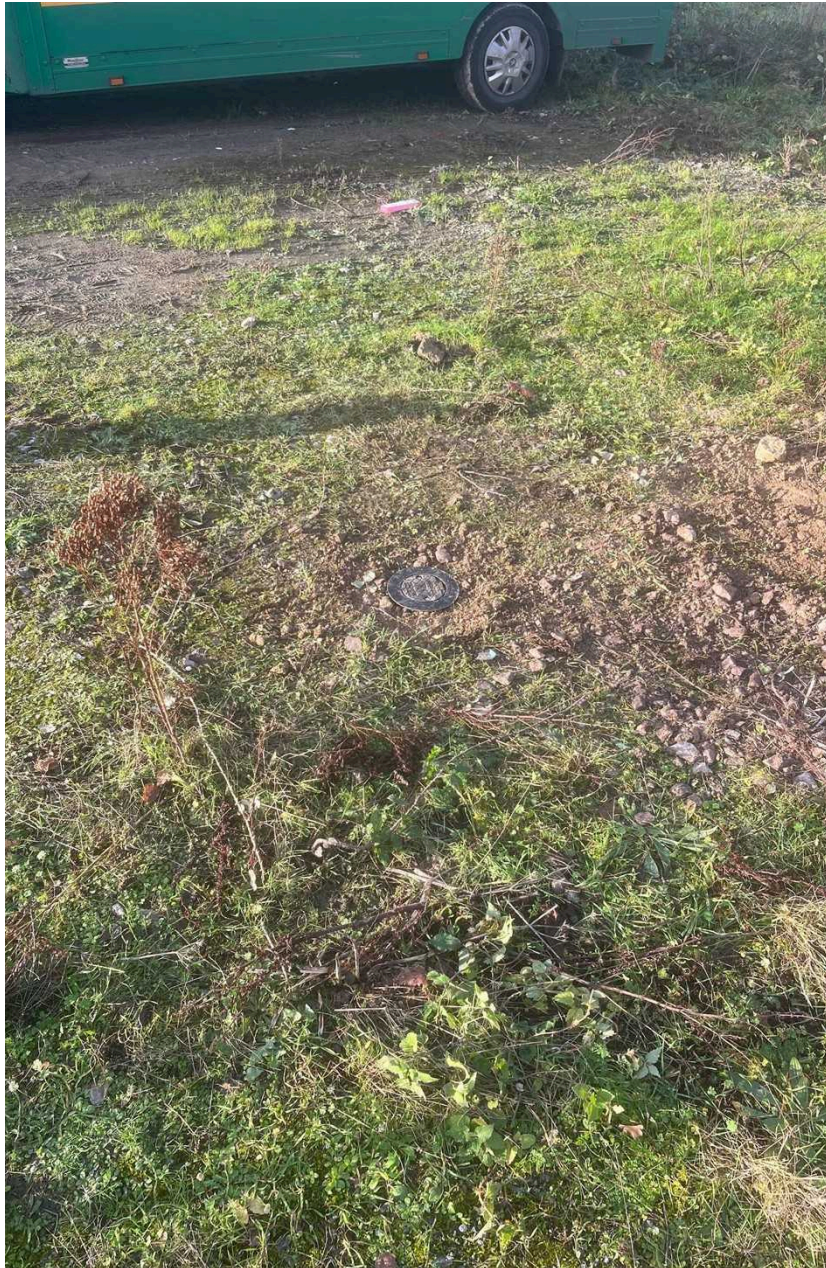
WS1 - Finished soakaway with flush cover
