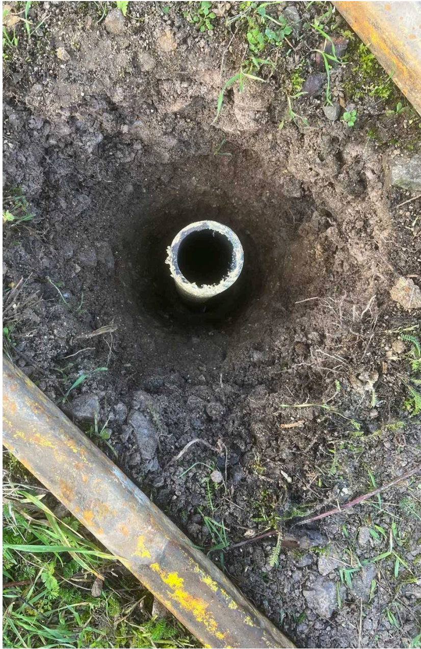
WS1 - with the fitted pipe
