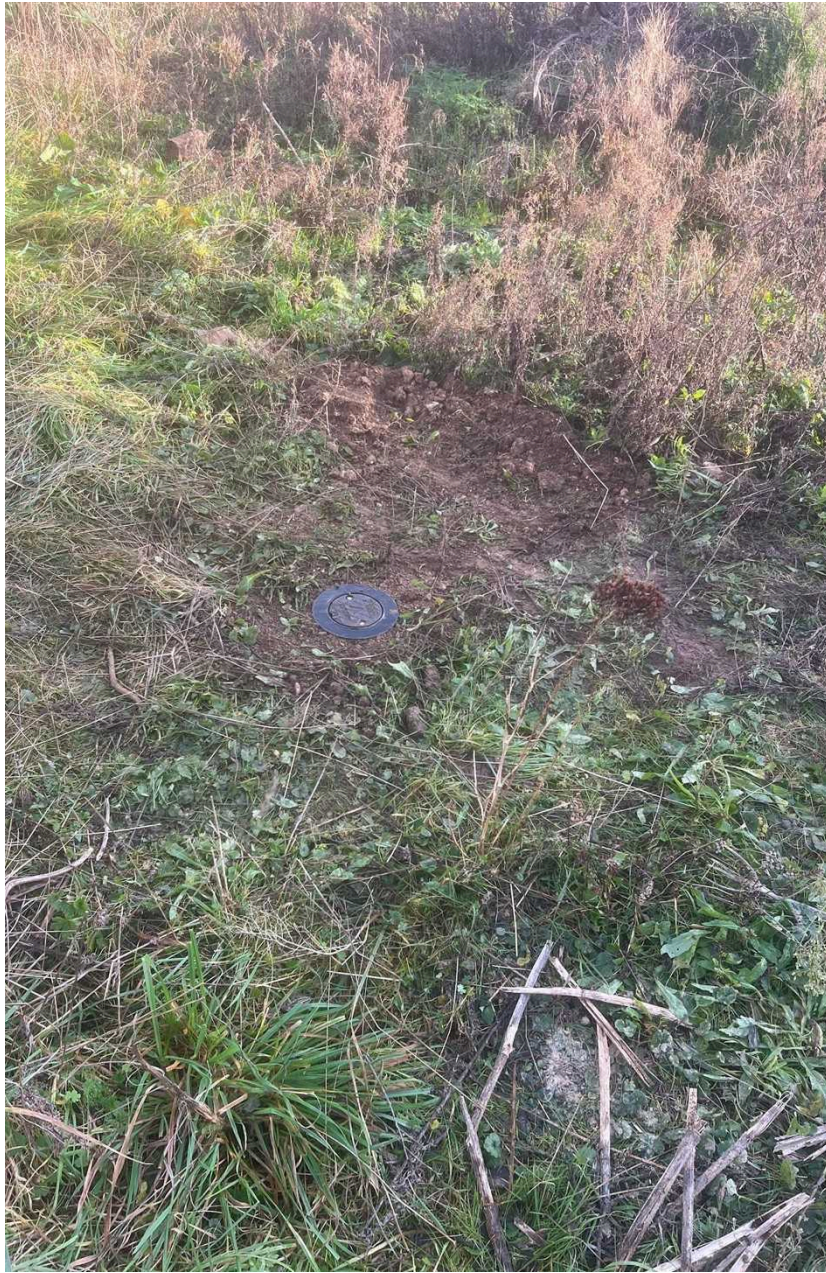
WS2 - Finished soakaway with flush cover
