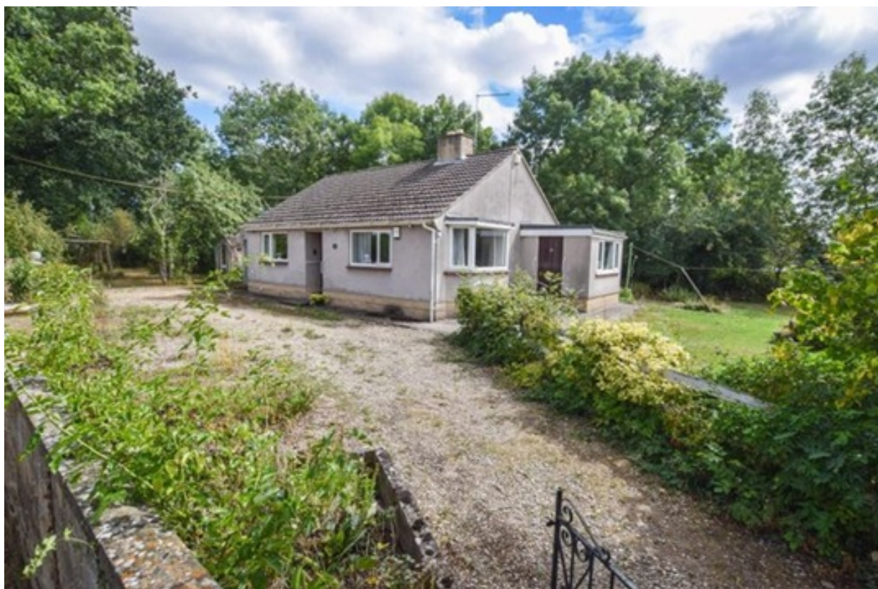
Existing frontage and side elevation facing north of The Haven, large gravel forecourt
