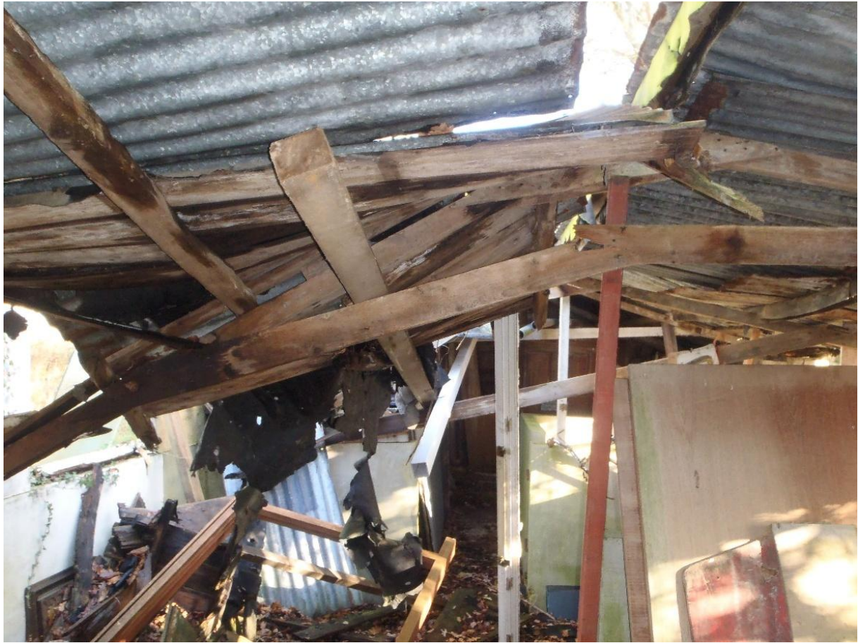
Photograph 9: showing an internal view of the former barn (Building 2)
