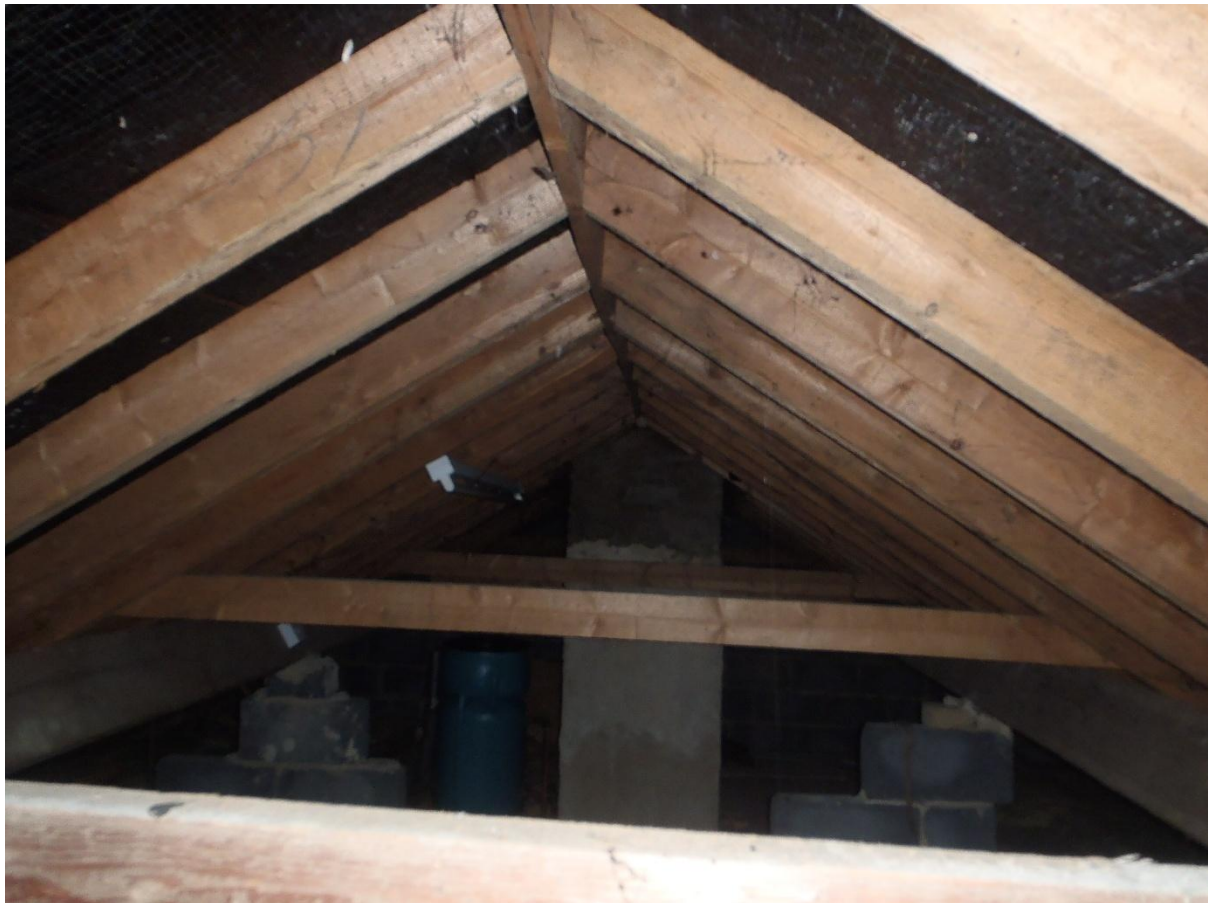
Photograph 6: showing a view of the loft space of the building (Building 1)
