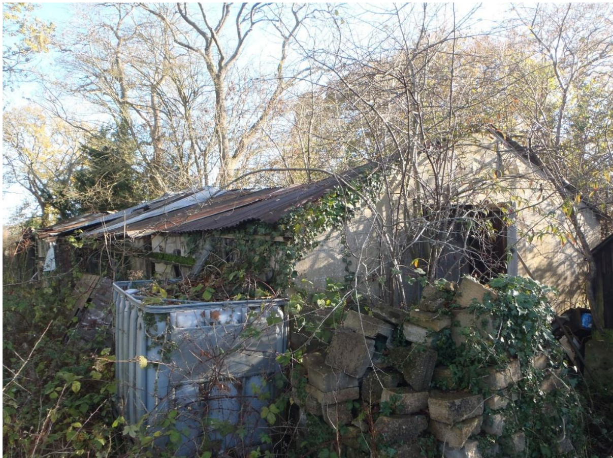
Photograph 8: showing a view of the former barn (Building 2)
