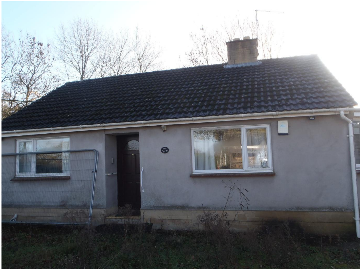
Photograph 5: showing a view of Building 1 (looking south)
