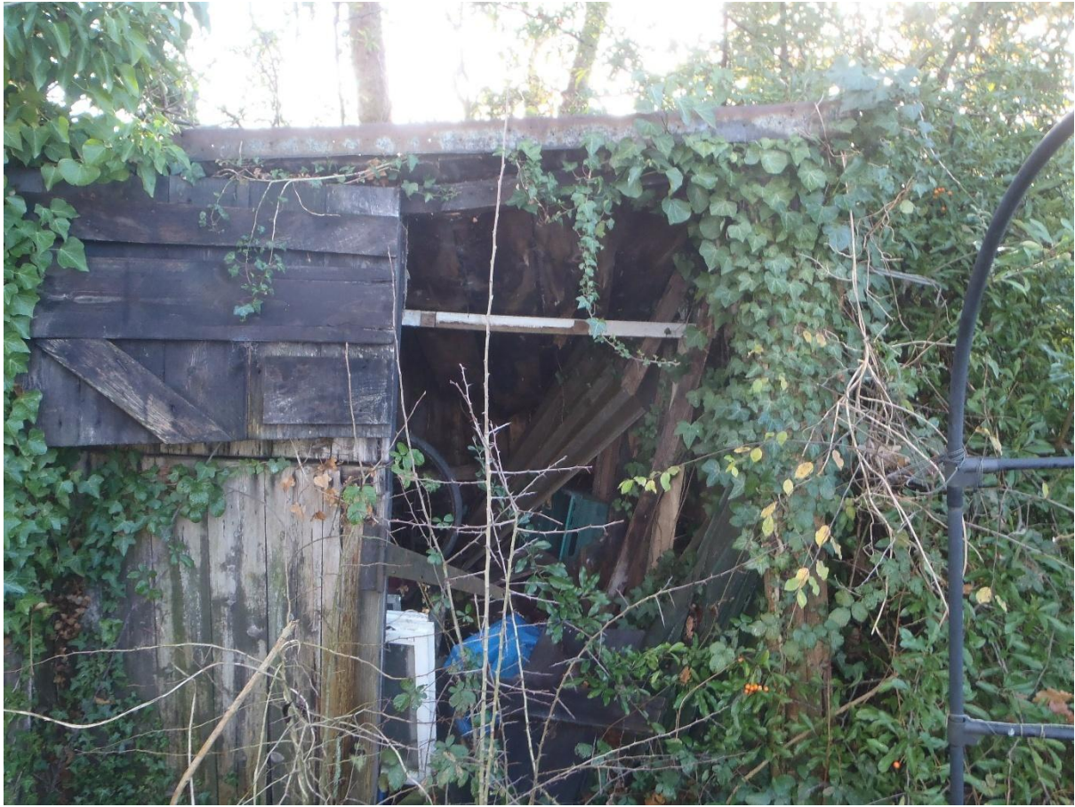
Photograph 10: showing a view of a shed outbuilding
