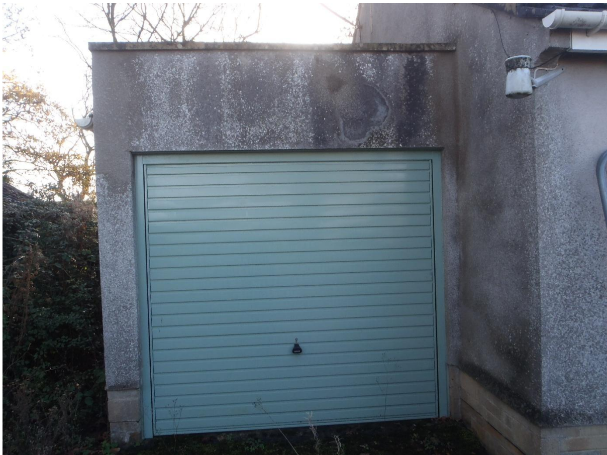
Photograph 7: showing a view of the garage building (adjacent to Building 1)
