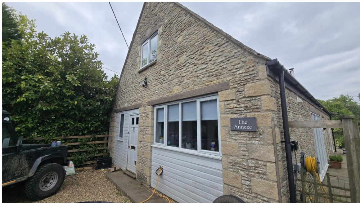
Fig. 1 – Principal Elevation of the Annexe
