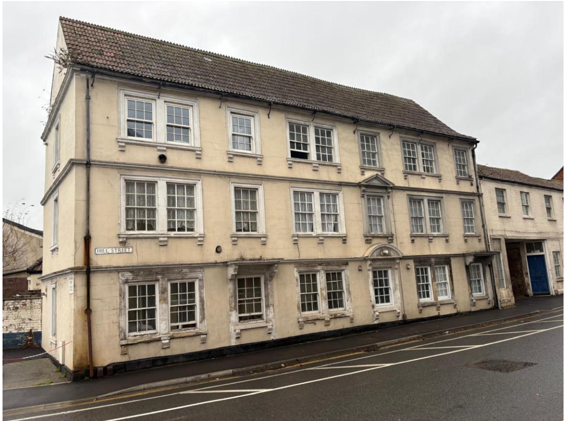
1. Kitchener's Court Front Elevation (East Facing)
