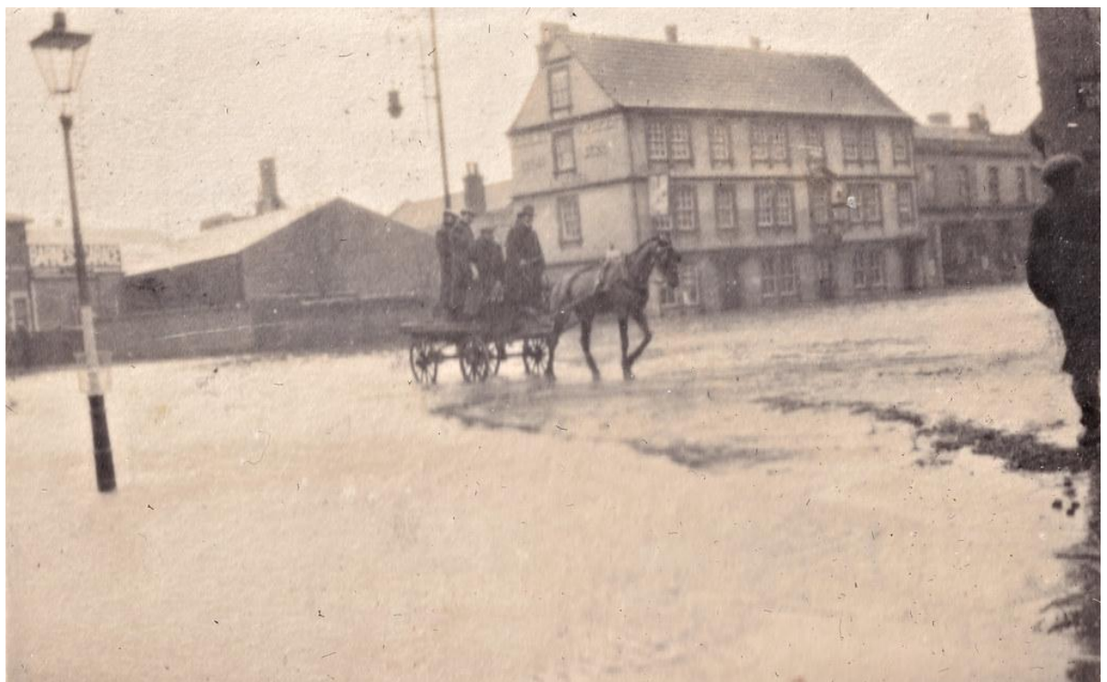
1916 Photograph showing flooding at Kitchener's Court – note there was once a window in the roof space.
