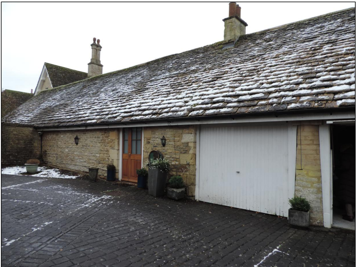
Photo 3 East facing view of the annex (northwest elevation) from within the courtyard.
