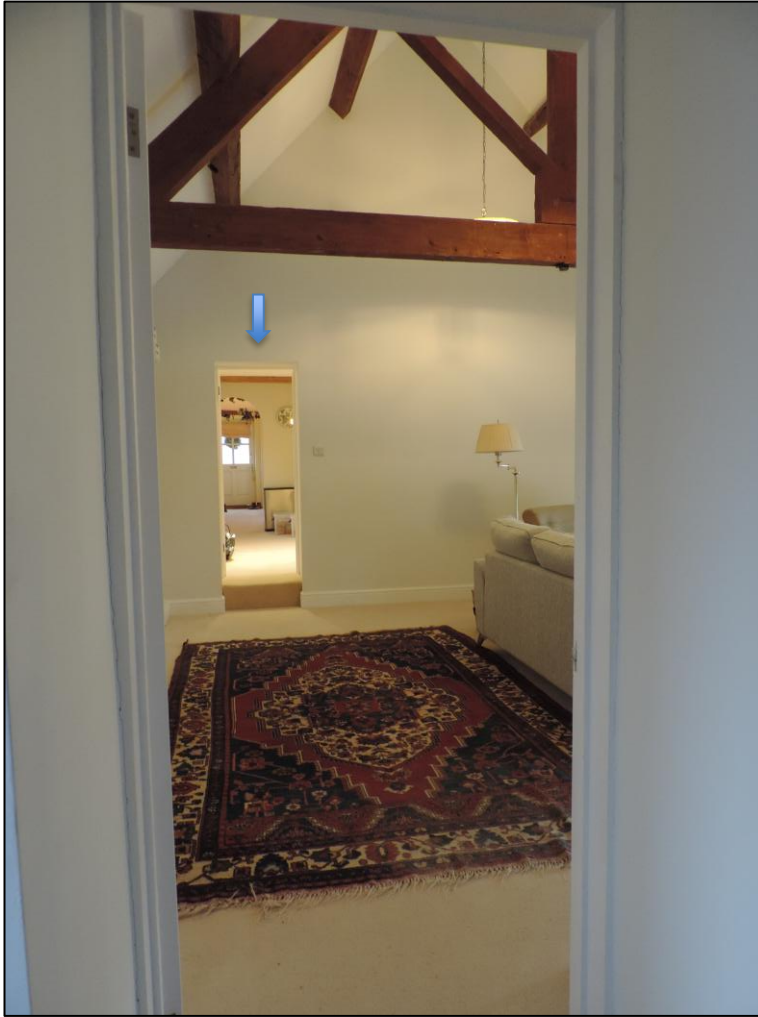
Photo 6 Northeast facing view of the knock through from the Hall to the Garden Room.
