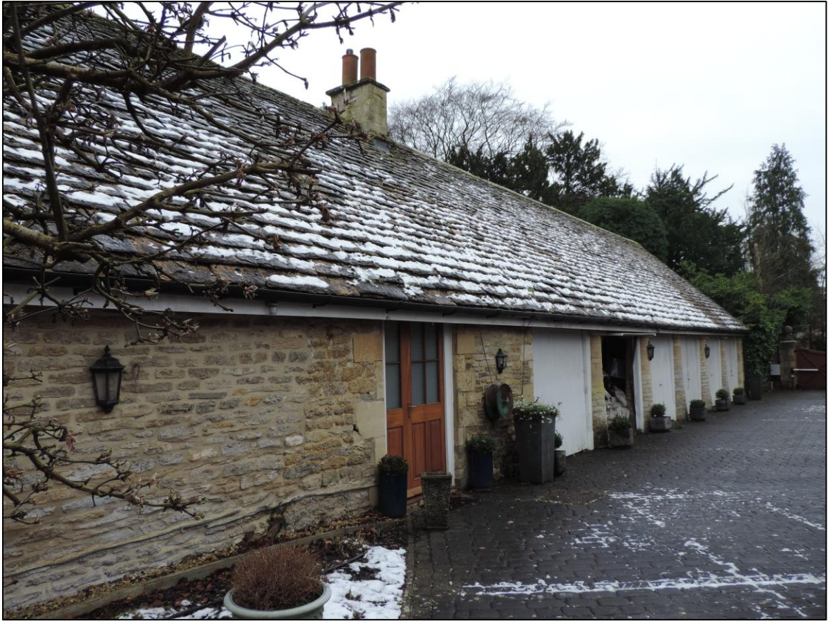
Photo 2 SSW facing view of southwest range (northwest facing elevation).
