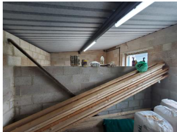
Photo 10: An internal view of building B2.
