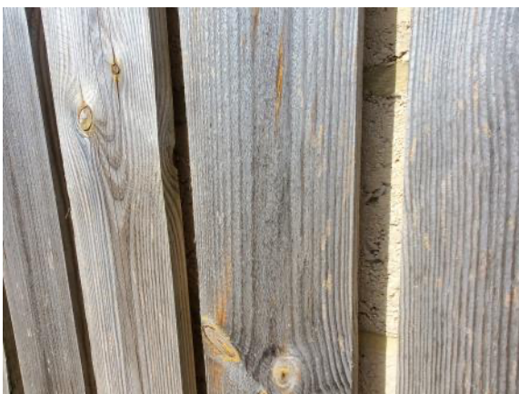
Photo 11: Timber cladding on the walls of B1 and B2.
