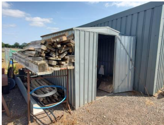
Photo 14: Building B4 viewed from the south.
