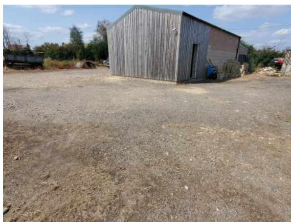
Photo 16: Gravelled surface which surrounds the buildings.
