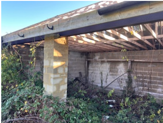
15: General interior view of the outbuilding.
