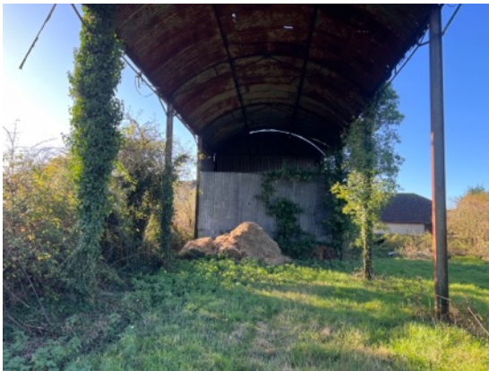
13: General interior of barn.
