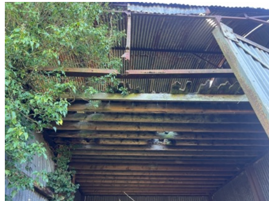
14: General interior of barn.
