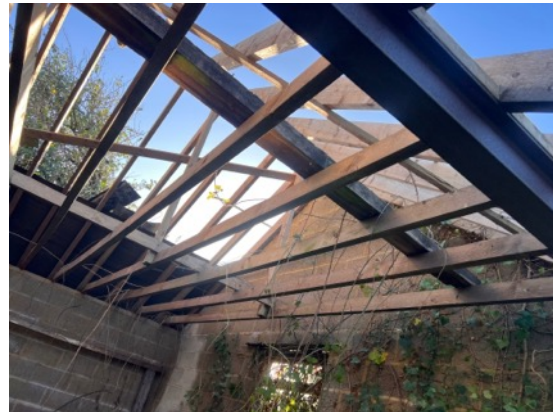
16: General interior view of the outbuilding.
