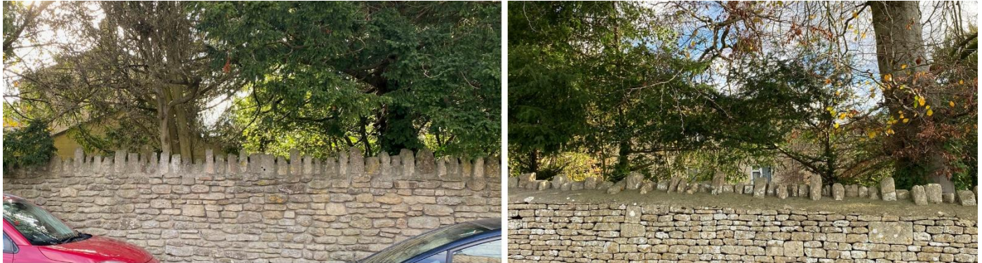
Site Visit External North and West Elevations
