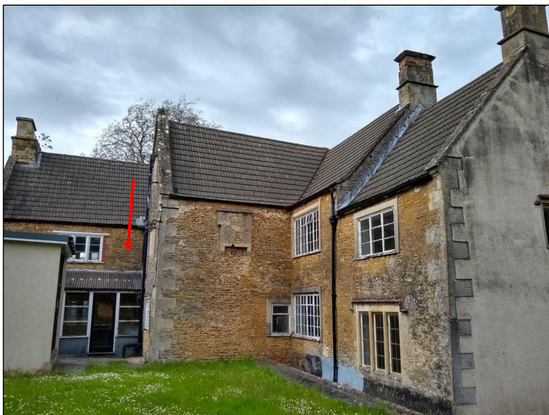
Photo 4 The western facing elements of the north-south range (lean-to arrowed)
