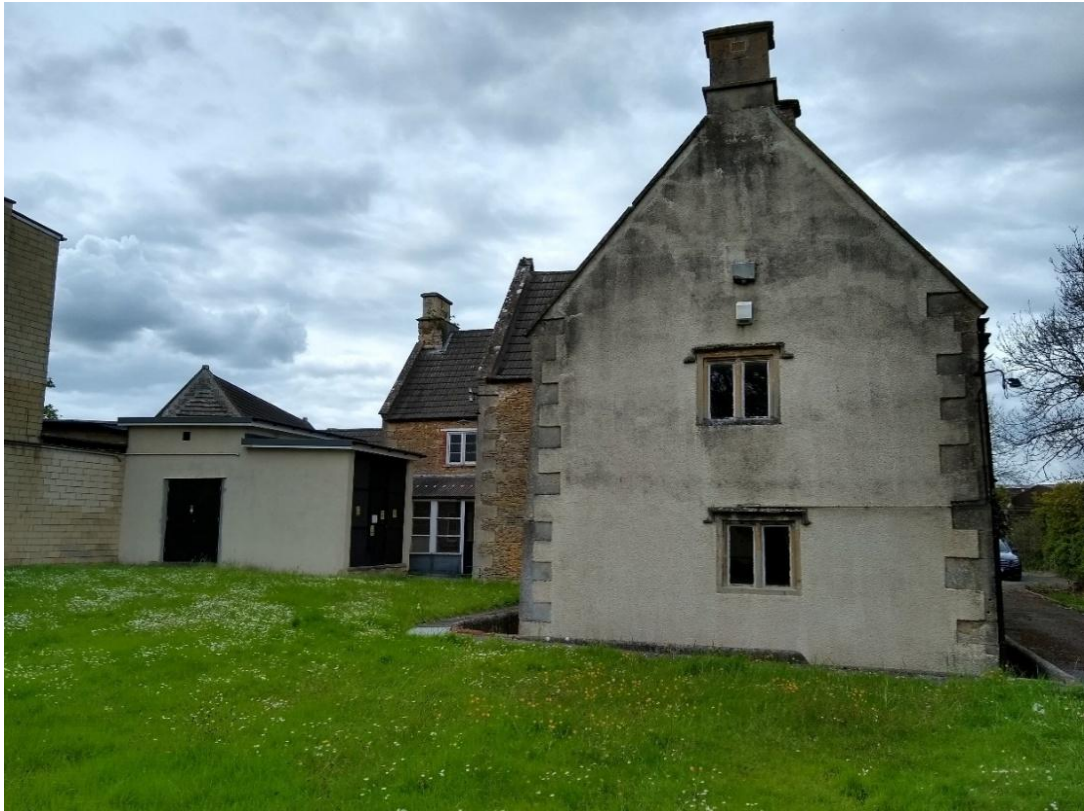
Photo 3 The south gable
