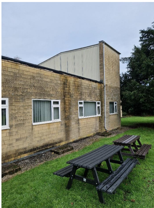
Photo 10 The south elevation of Extension 1
