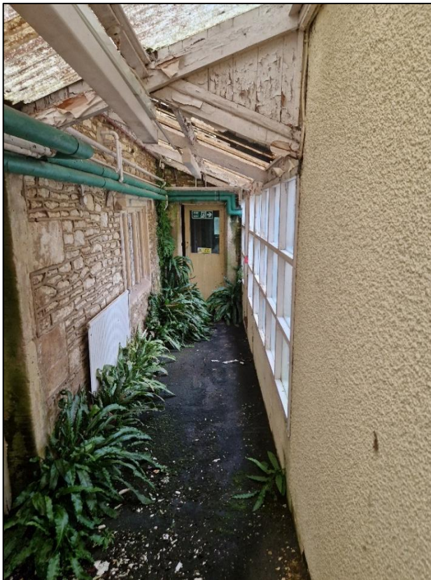
Photo 13 Interior of the lean-to to removed
