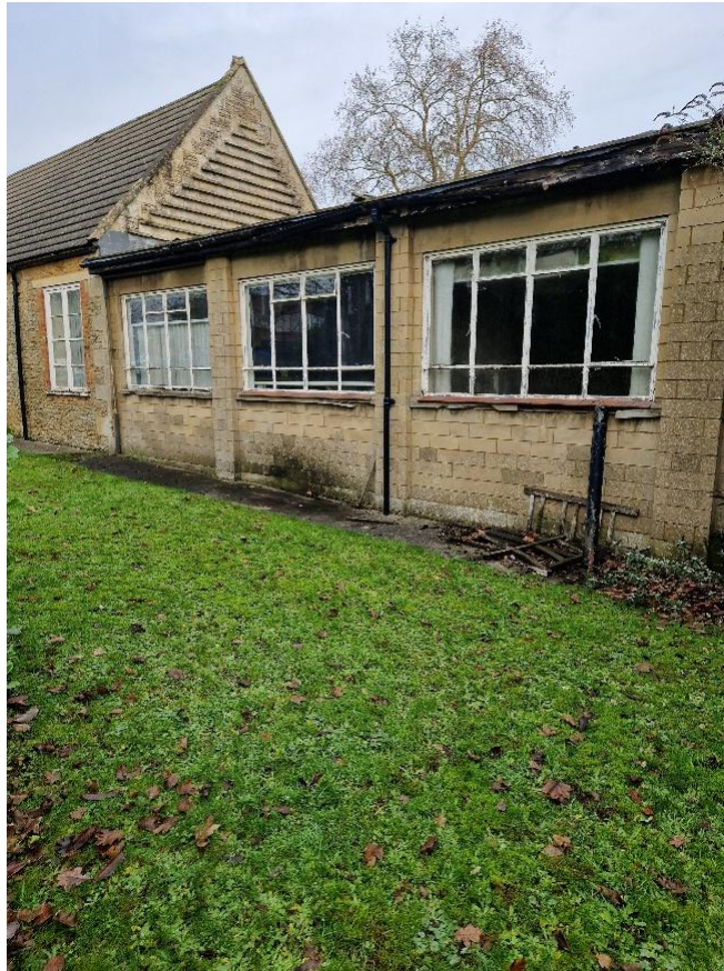
Photo 15 The west elevation of Extension 3 abutting the south gable of the barn
