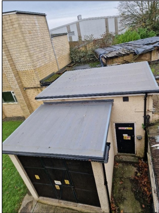
Photo 11 Extension 2 seen from a first-floor window
