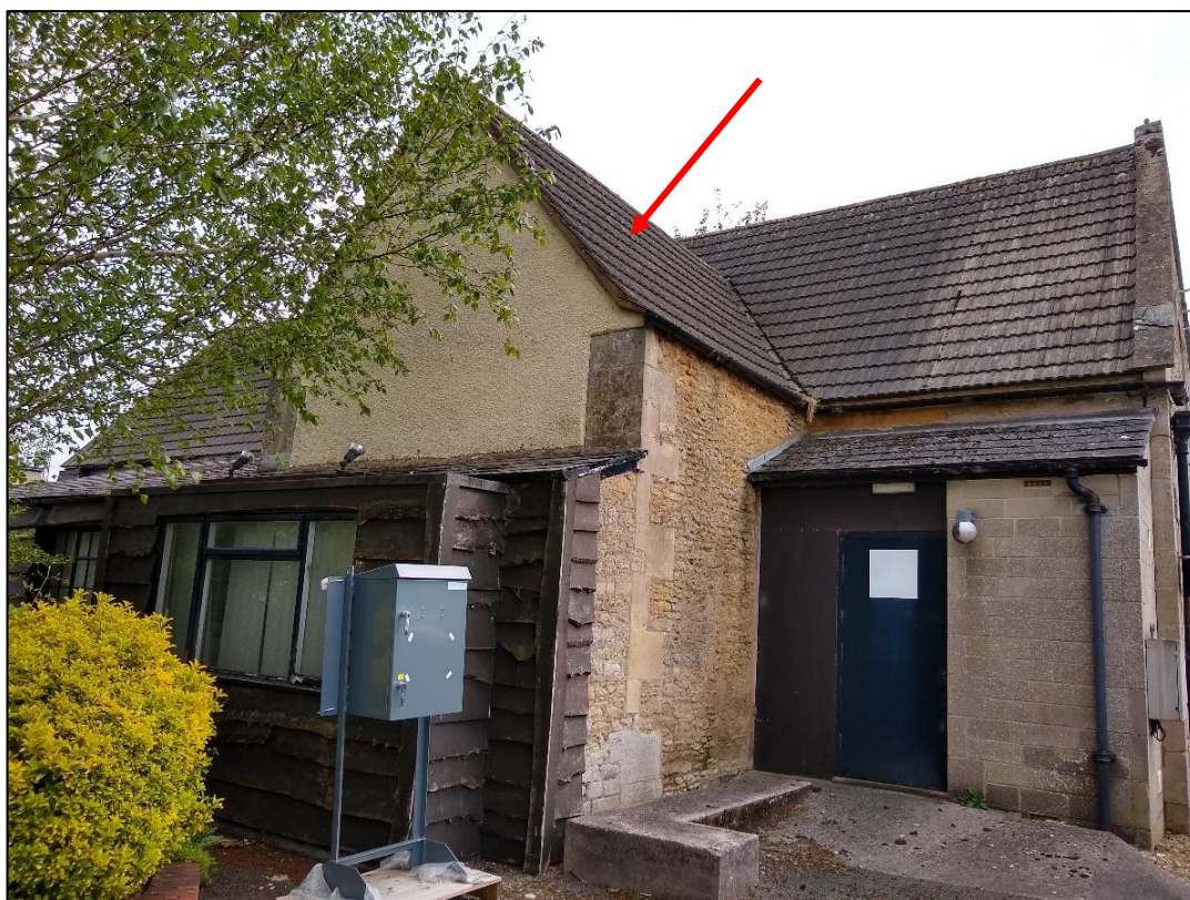
Photo 6 The former barn with additions over the former threshing porch (arrowed)
