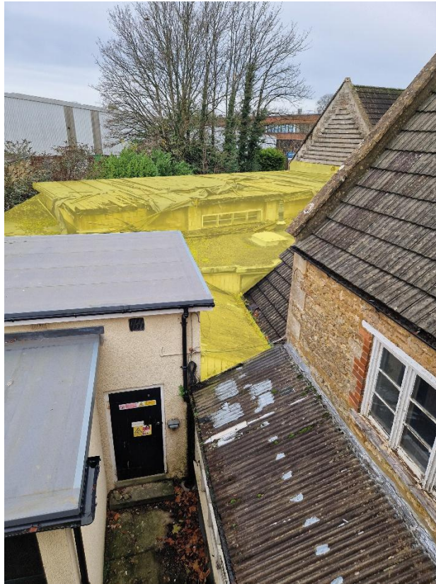
Photo 12 Image of roofscape depicting Extension 3
