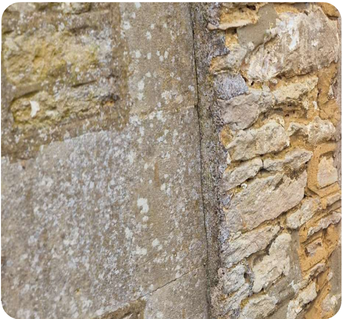
STONE QUOINS REINSTATED
