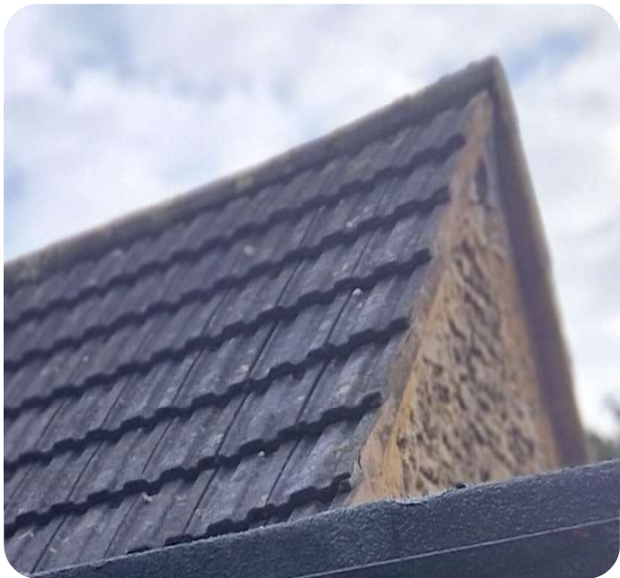
MORTAR BEDDED VERGE DETAIL
