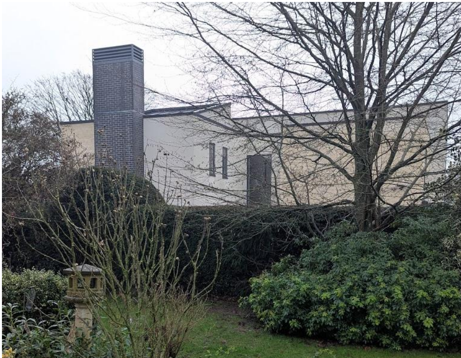
View From No 44 Neighbour of Existing western elevation
