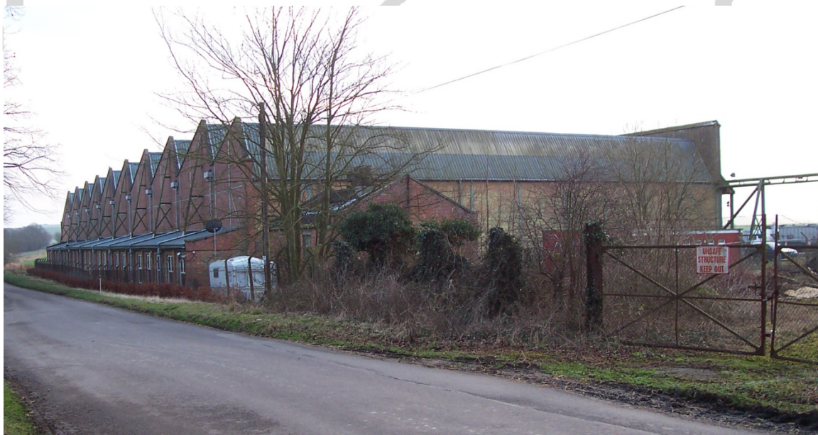
Hangar 45 2005 before restoration works. Image: geograph.org.uk
