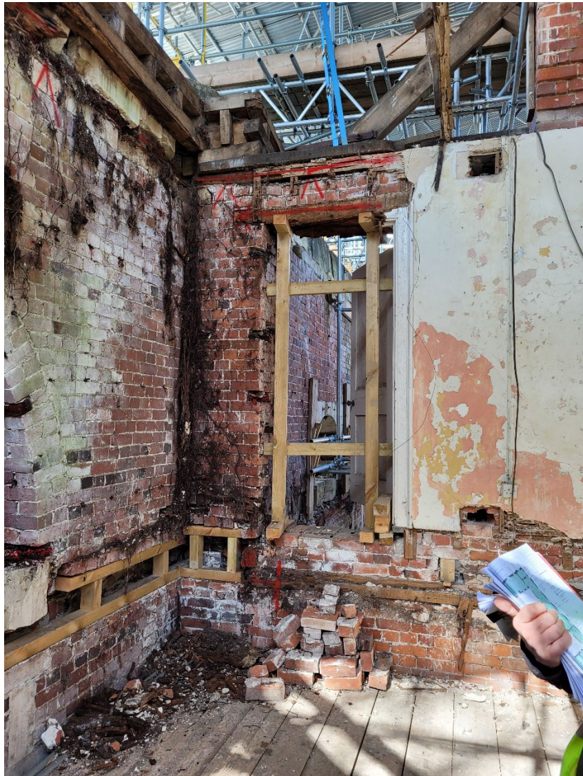
Image 2 – Existing fabric at First Floor
