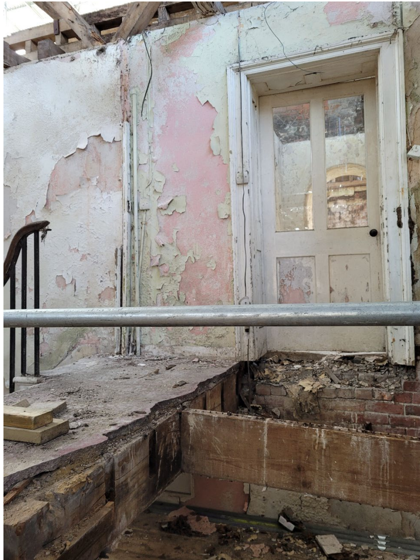
Image 1 – Existing fabric at First Floor
