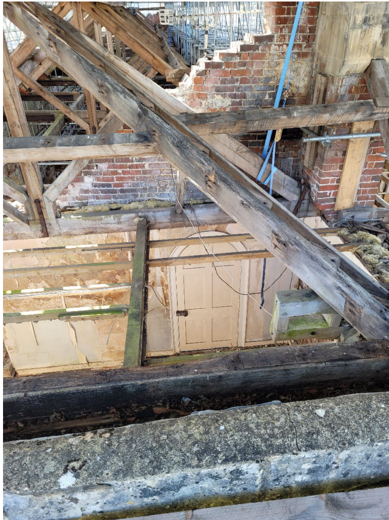
Image 3 – Existing fabric at First Floor
