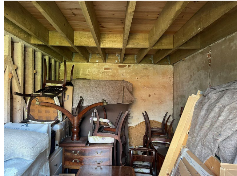
Plate 21: 'Garage' portion of the Coach House.
