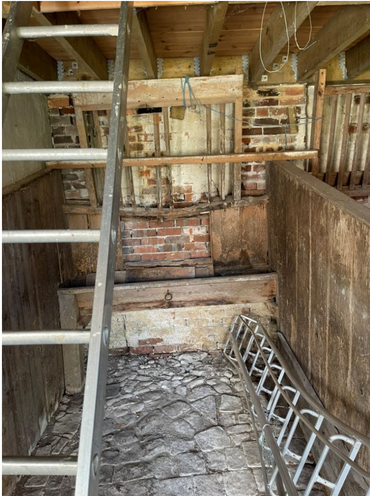
Plate 20: View of cobble flooring and interior fittings of the ground floor of the Coach House.
