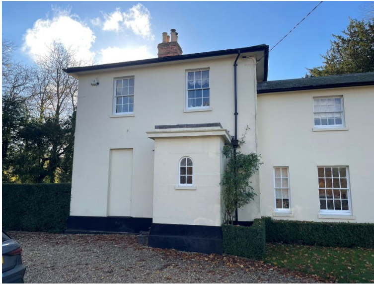
Plate 10: The northern elevation of the hipped roof section of the house.
