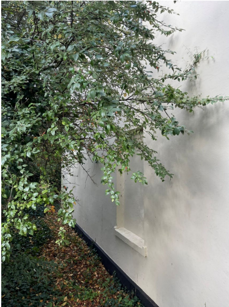
Plate 14: Closeup of the southern elevation of the bay wing.
