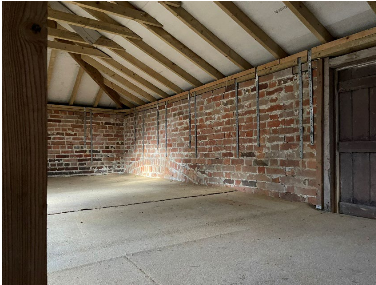
Plate 19: View of the attic floor of the coach house.
