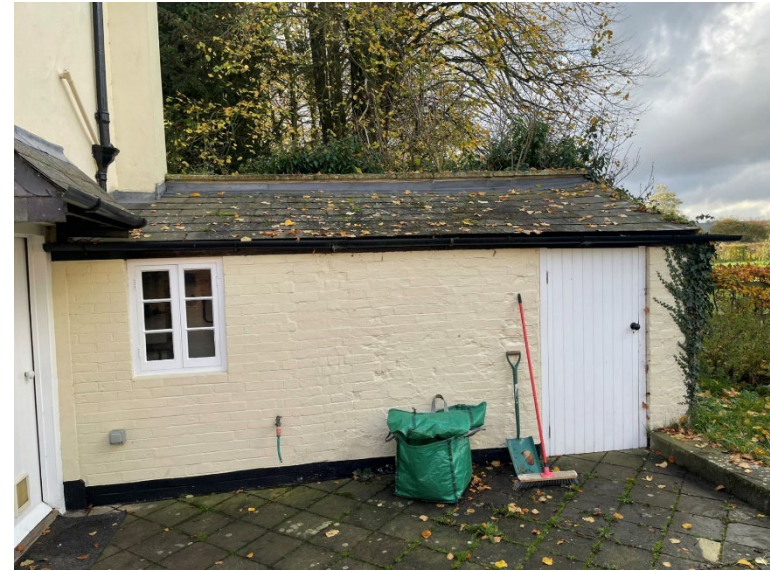
Plate 15: Northern elevation of the western projecting range.
