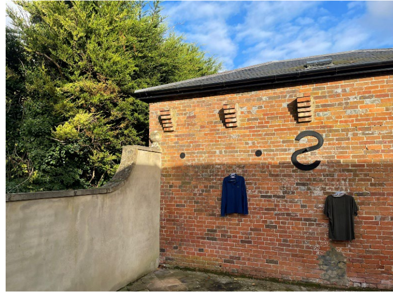
Plate 18: Southern elevation of the Coach House; showing the court feature.
