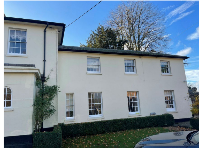
Plate 11: The fenestration of the northern elevation's bay wing.
