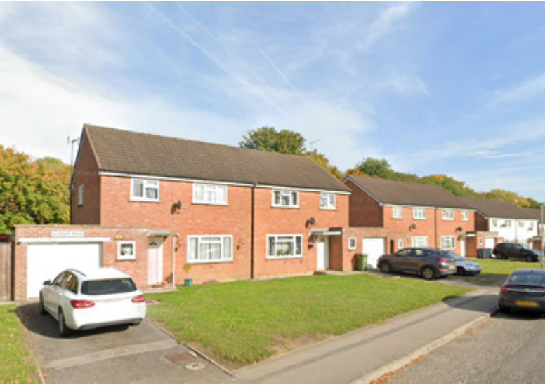
Photo: Houses on Slessor Road, Lyneham
