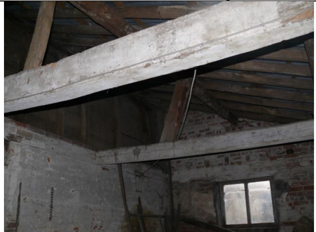
Western interior of building 2
