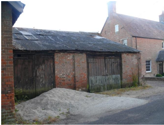
Northern elevation of building 2
