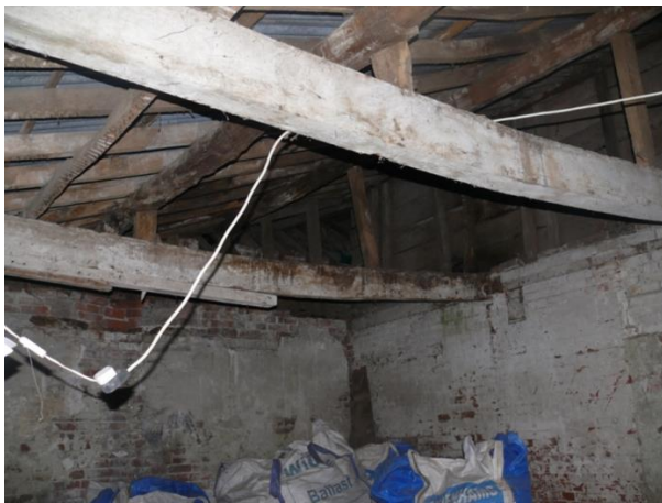
Eastern interior of building 2
