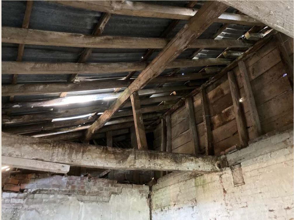
Figure 9: Roof structure of Tractor shed
