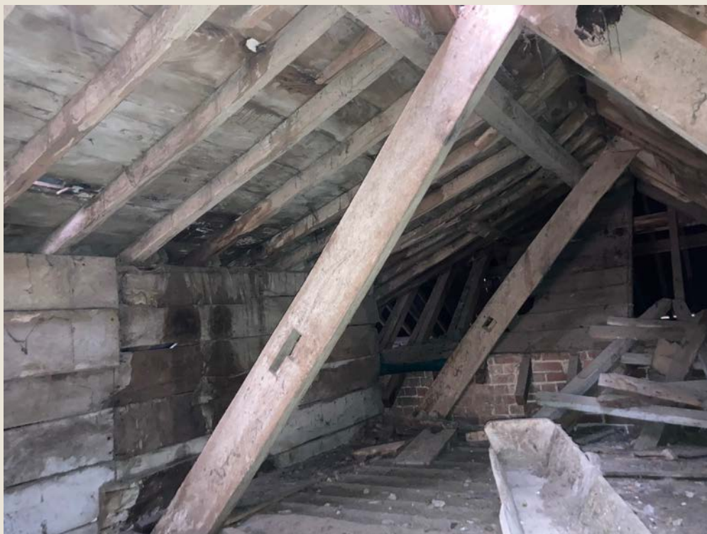
Figure 15: Stable 1 roof structure
