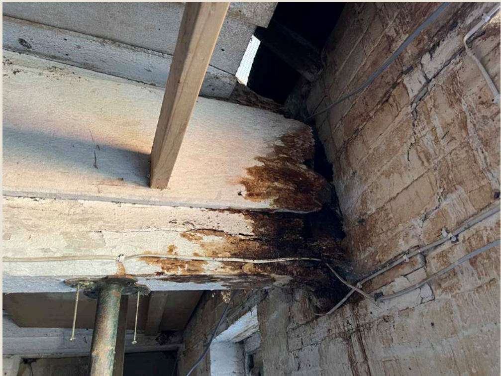
Figure 12: Stable 1 interior, concrete floor
