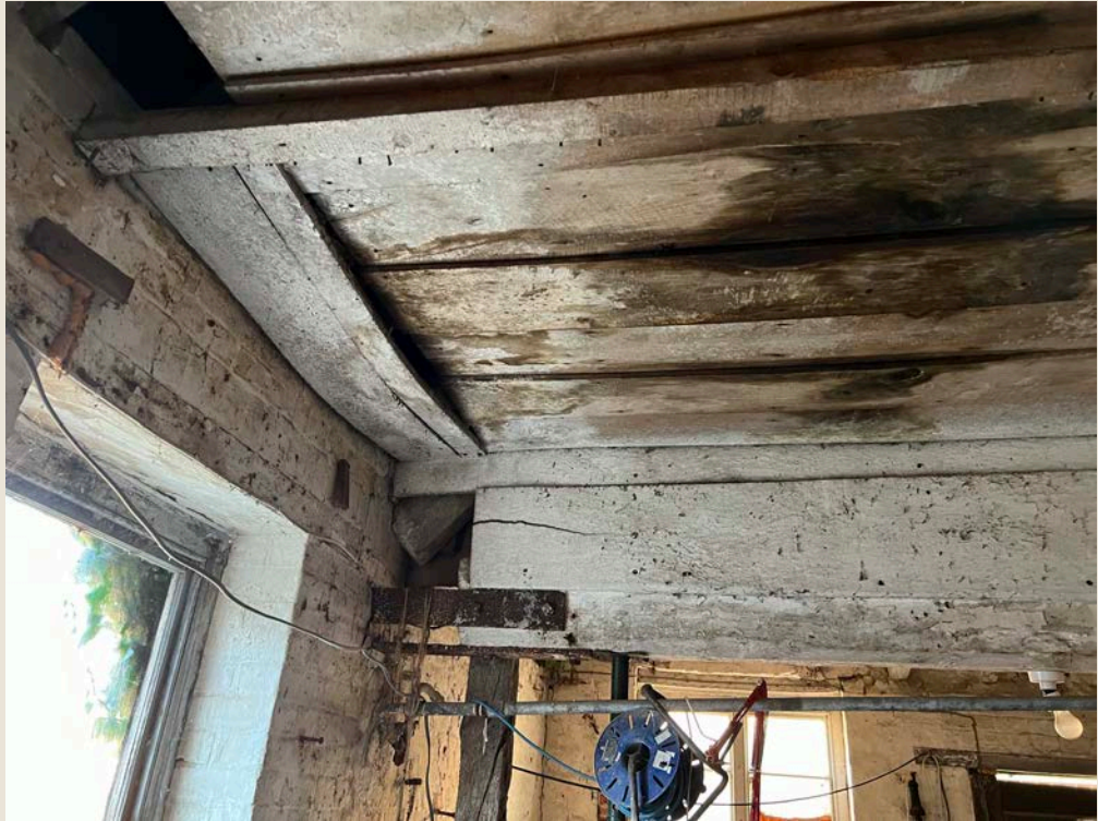
Figure 11: Stable 1 interior, showing propped beam
