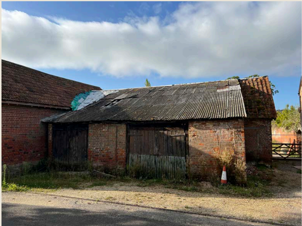
Figure 2: North elevation of Tractor shed from road
