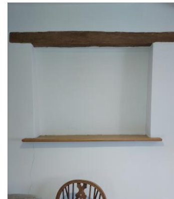
Door Opening in 2026 - bottom half of door has been filled in to form opening for a future window
