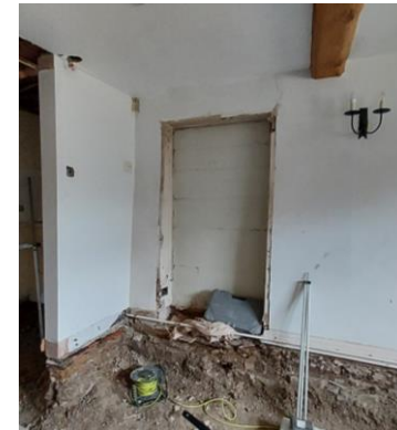
Original door opening exposed during renovations in 2024
