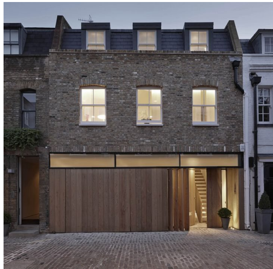
Above left: Lightweight timber link. Above right: Street front cladding and clerestory windows.
