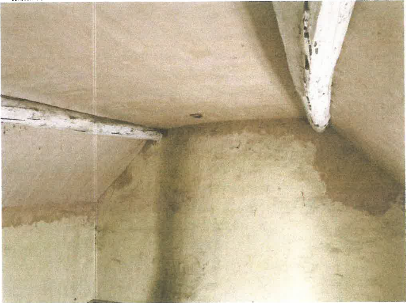
Figure 2 - Ceiling present to western half of original roof
