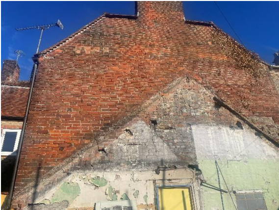
Before Rear Elevation – Top
