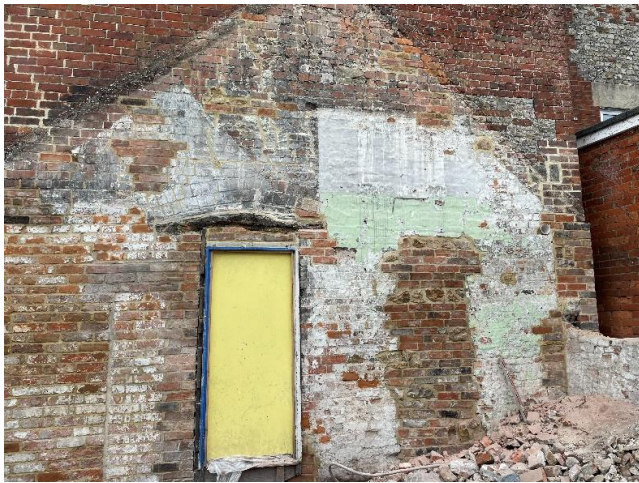
After Rear Elevation -RHS
