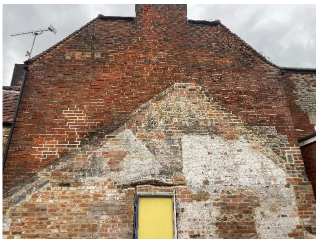
After Rear Elevation – Top 2
