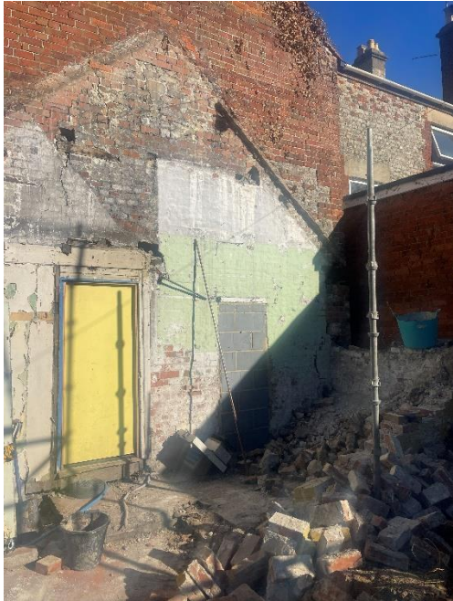
Before Rear Elevation - RHS
