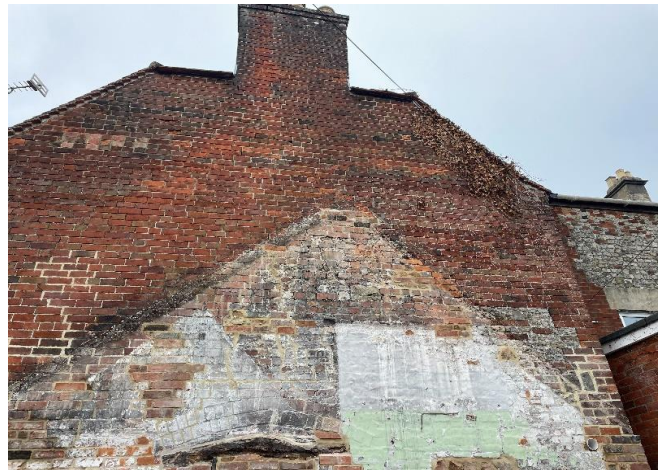
After Rear Elevation – Top 1
