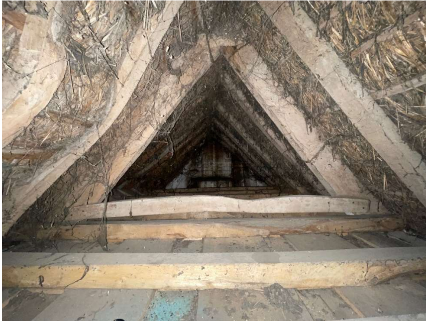
Fig 4.0 photograph of existing roof space (looking NE)
