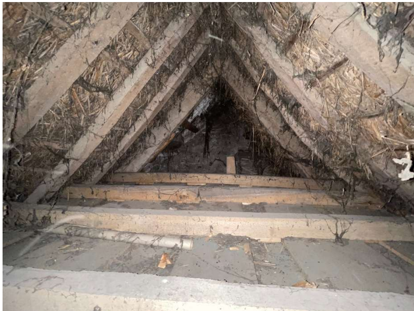
Fig 5.0 photograph of existing roof space (looking SE)
