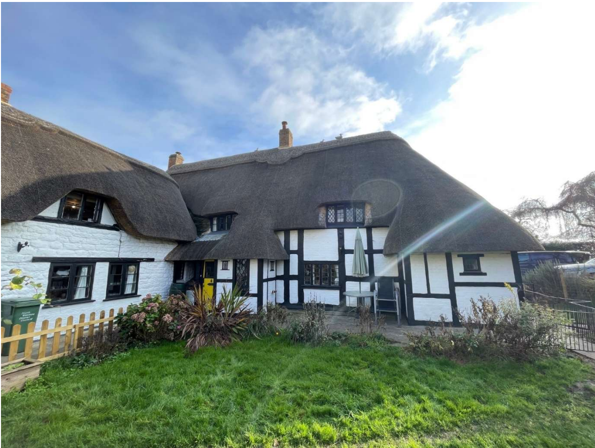
Fig 3.0 photograph of north west elevation
