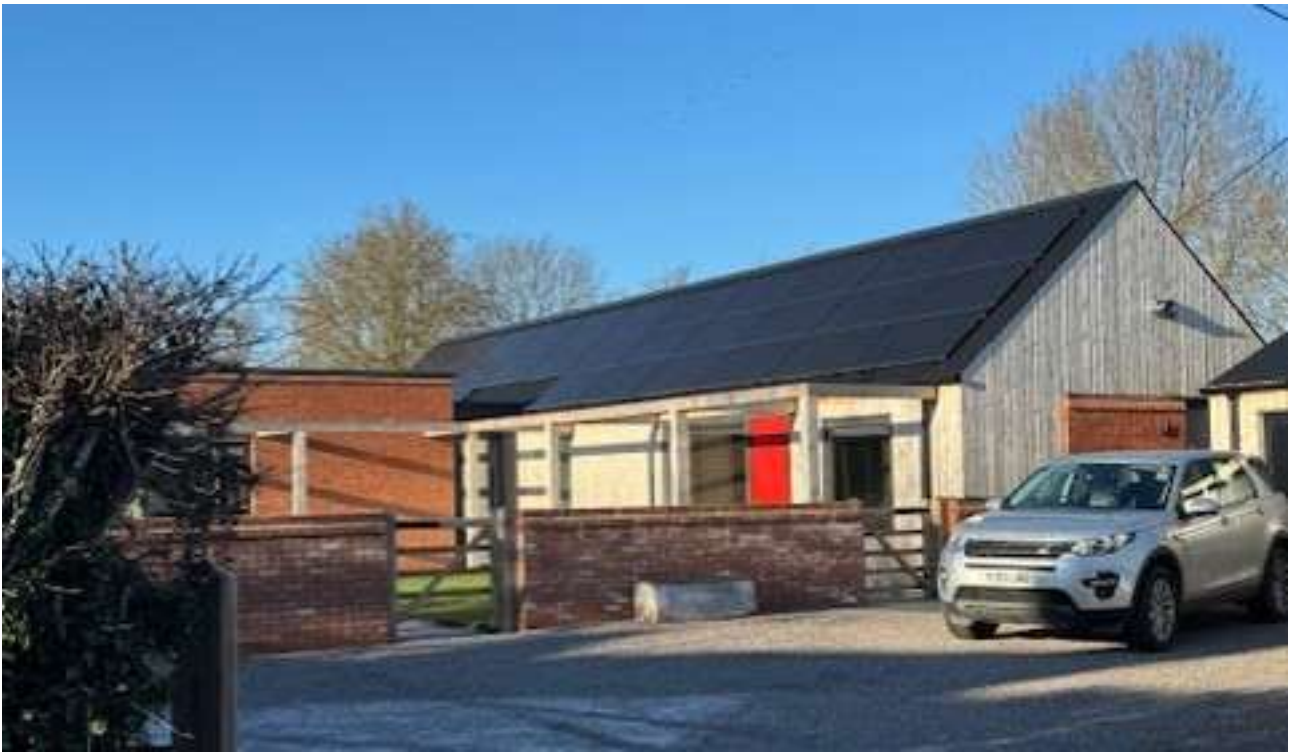
Fig 3.3 photograph of new build house with PV array
