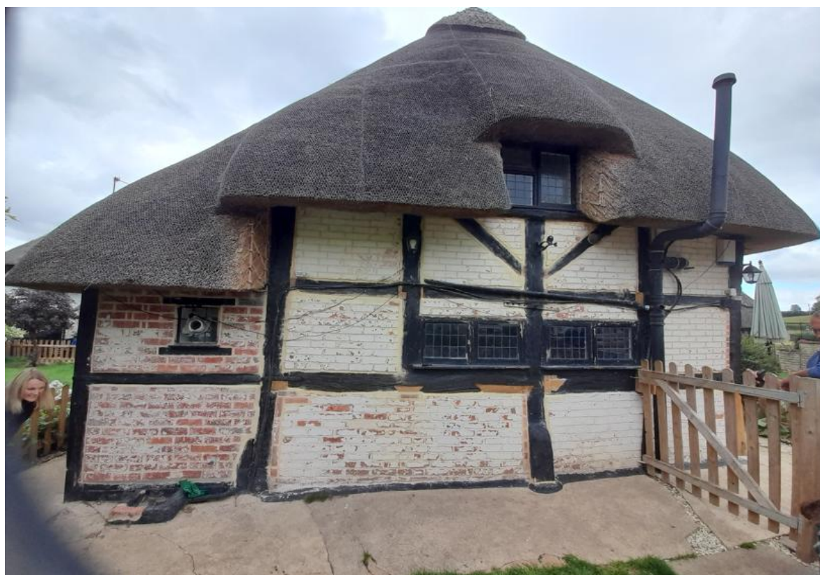
Fig. 10: View, looking north, of the south-west, end elevation of the north-east/south-west range.
