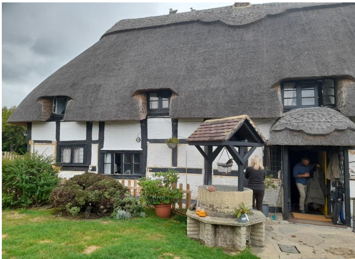
Fig. 11: View, looking west, of the left-hand side of the south-east elevation of the north-east/south-west range.
