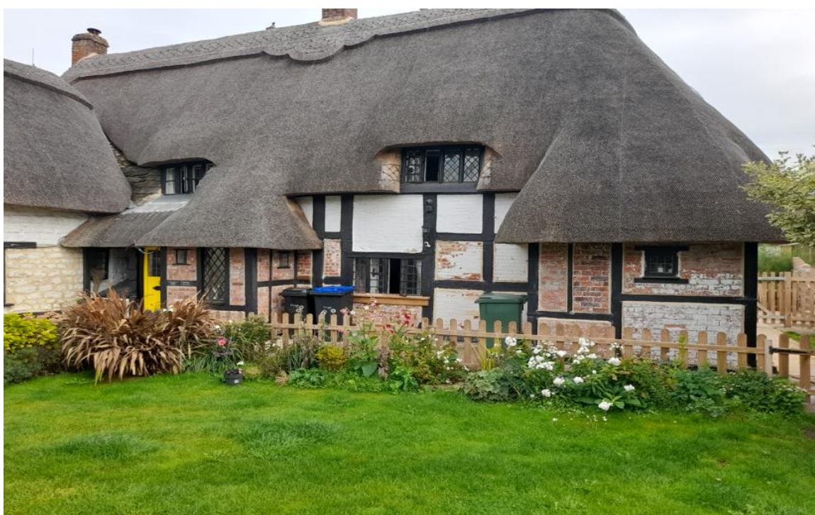
Fig. 7: View, looking north-east, of the south-west elevation of the north/west/south-east range.
