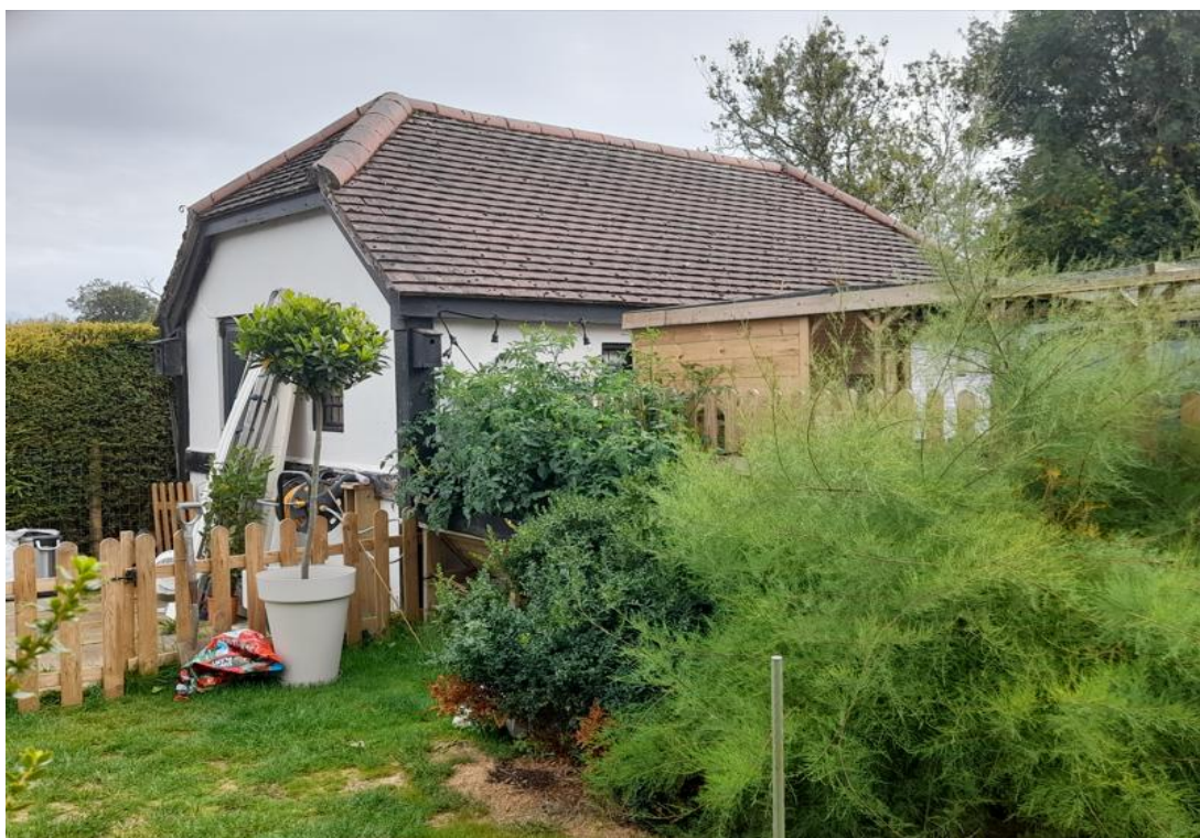
Fig. 36: View of the north-eastern end of the existing garage, looking west.
