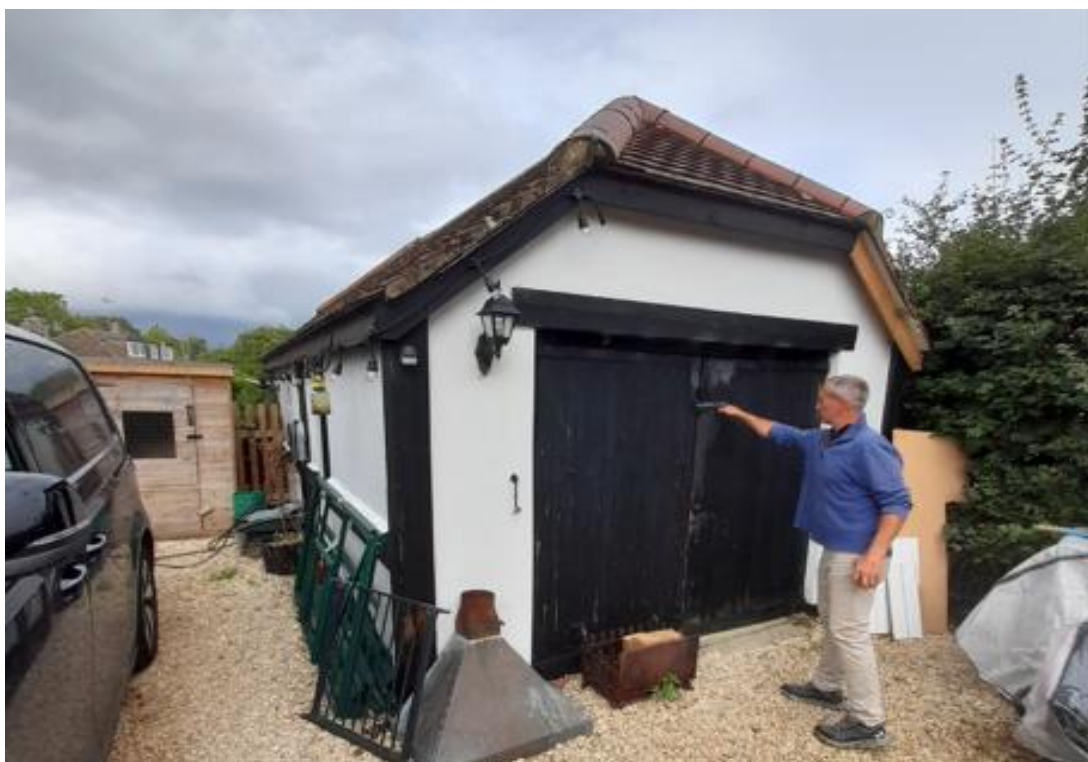
Fig. 37: View of the south-western end of the garage, looking north-east.
