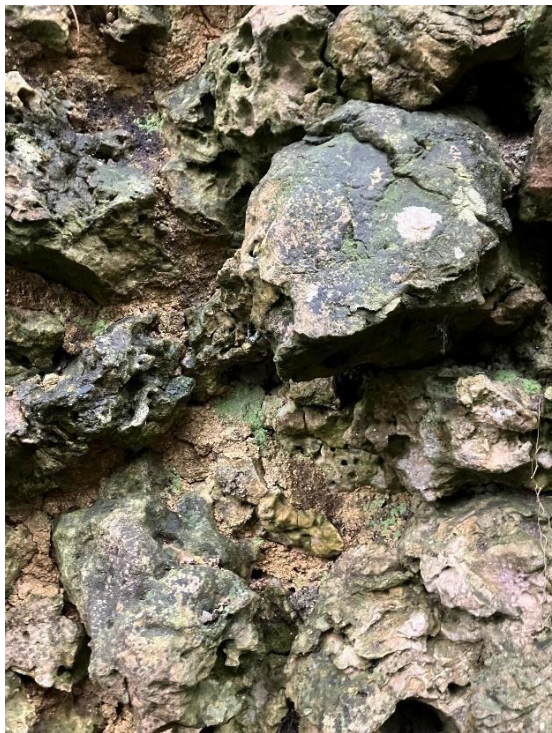
Fig 7: Tufa stone facing bedding mortar.
