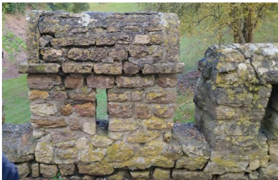
Fig 12: Merlon cappings to be rebuilt.
