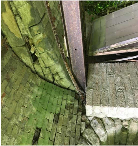
Fig 14: Block and steel beam support to be removed.
