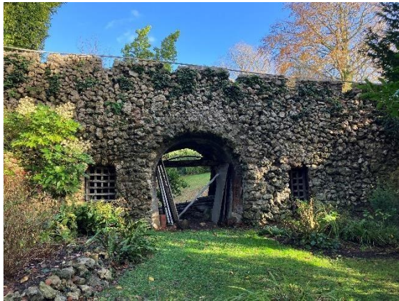
Fig 5: Moat Bridge West Elevation.
