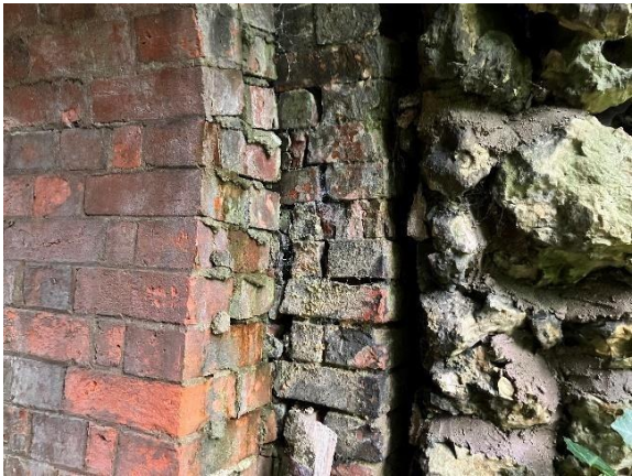
Fig 6: Brickwork to south side of Arch 2.
