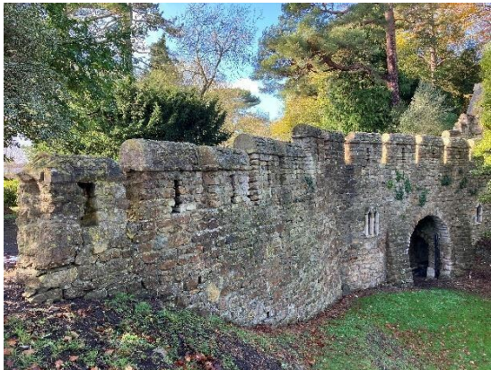
Fig 1: Moat Bridge East Elevation
