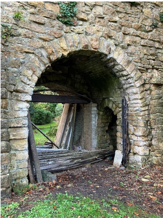
Fig 3: Arch 1 with doorway to Chamber 1
