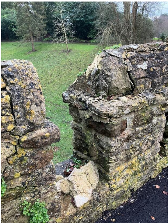
Fig 8: Hard Cement parapet pointing.
