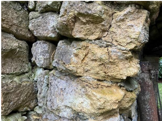
Fig 2: Left side of Arch 1
