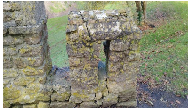
Fig 13: Merlon cappings to be rebuilt
