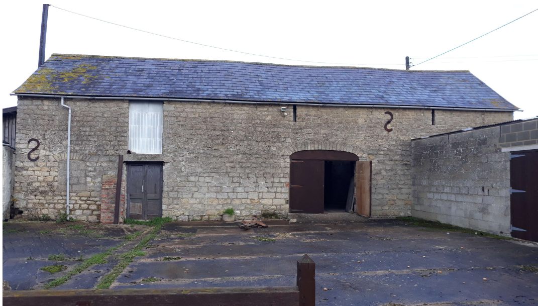
View of the stone barn, looking north.
