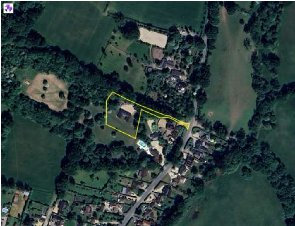
Figure 1 - Aerial view of application site
