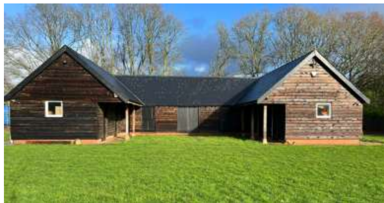
Figure 8 - Existing south elevation
