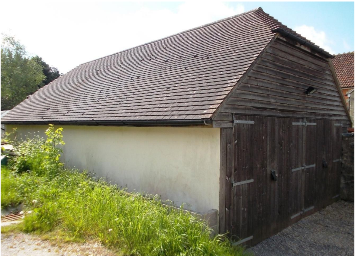
Fig 3.2b; view of north and west elevations
