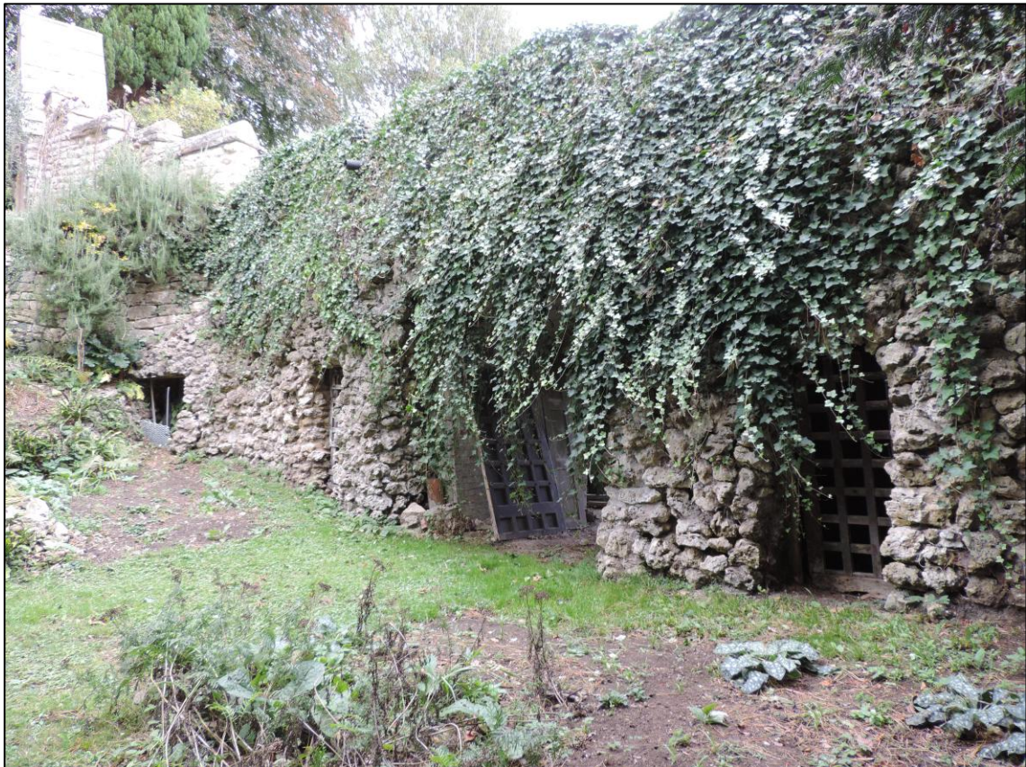
Photo 2 North facing view of Moat Bridge, southwest elevation.
