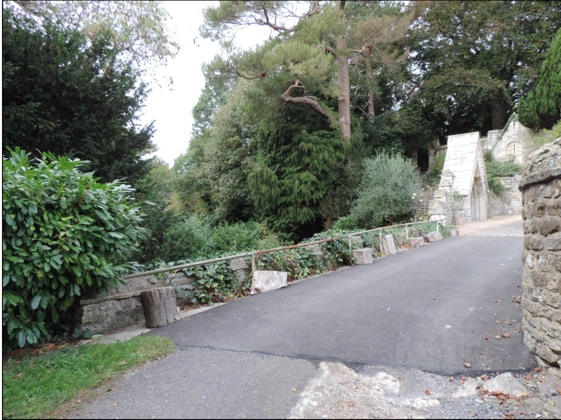
Photo 3 Northwest facing view of bridge deck, with low parapet and guard rail visible on SW side.
