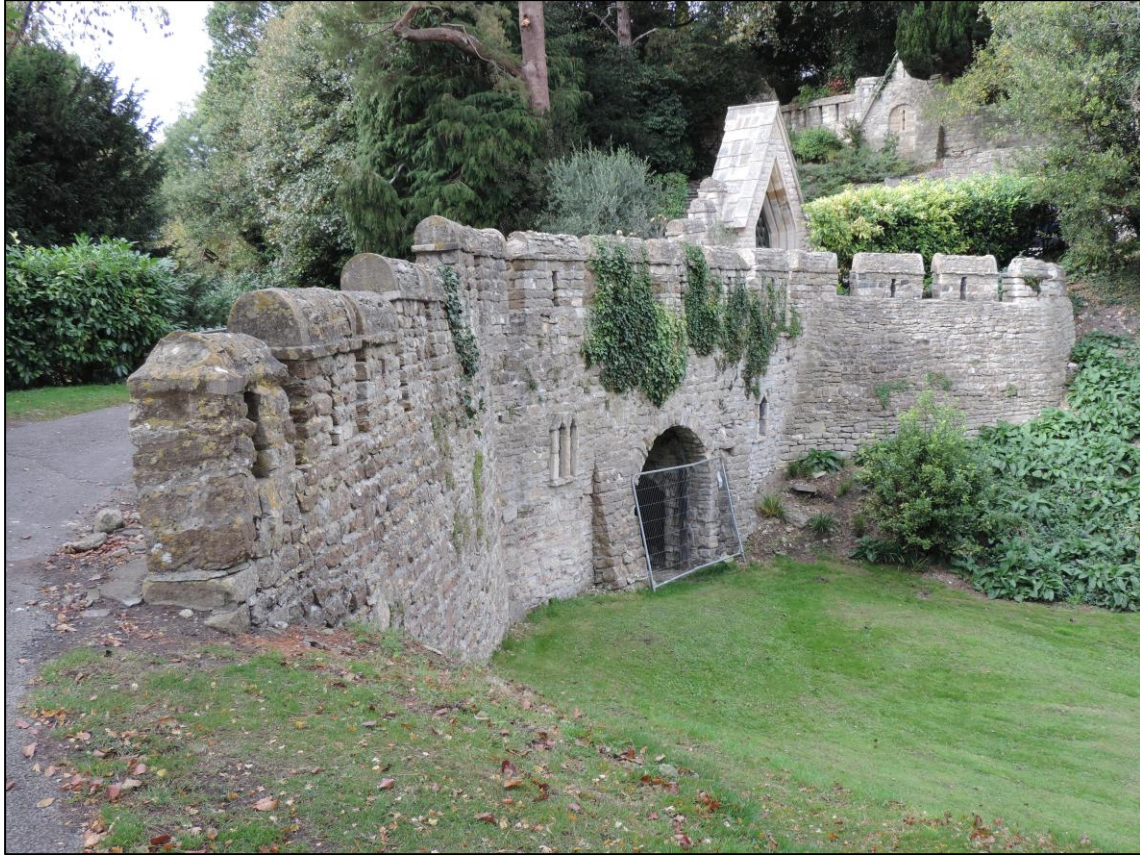
Photo 1 Northwest facing view of Moat Bridge, northeast elevation.
